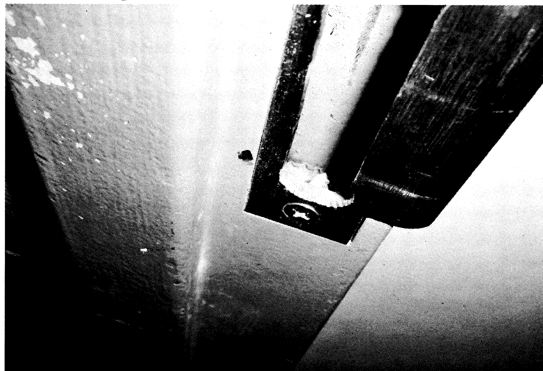
After living with a broked door, the door jam is drilled out to fit a temporary one.
