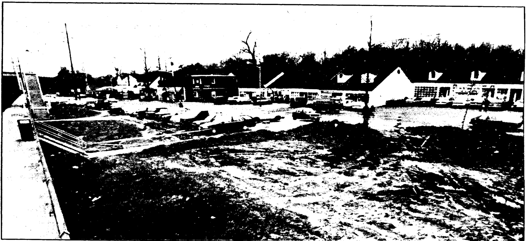
Construction has already begun in the area North of the railroad station preventing cars from parking there.
