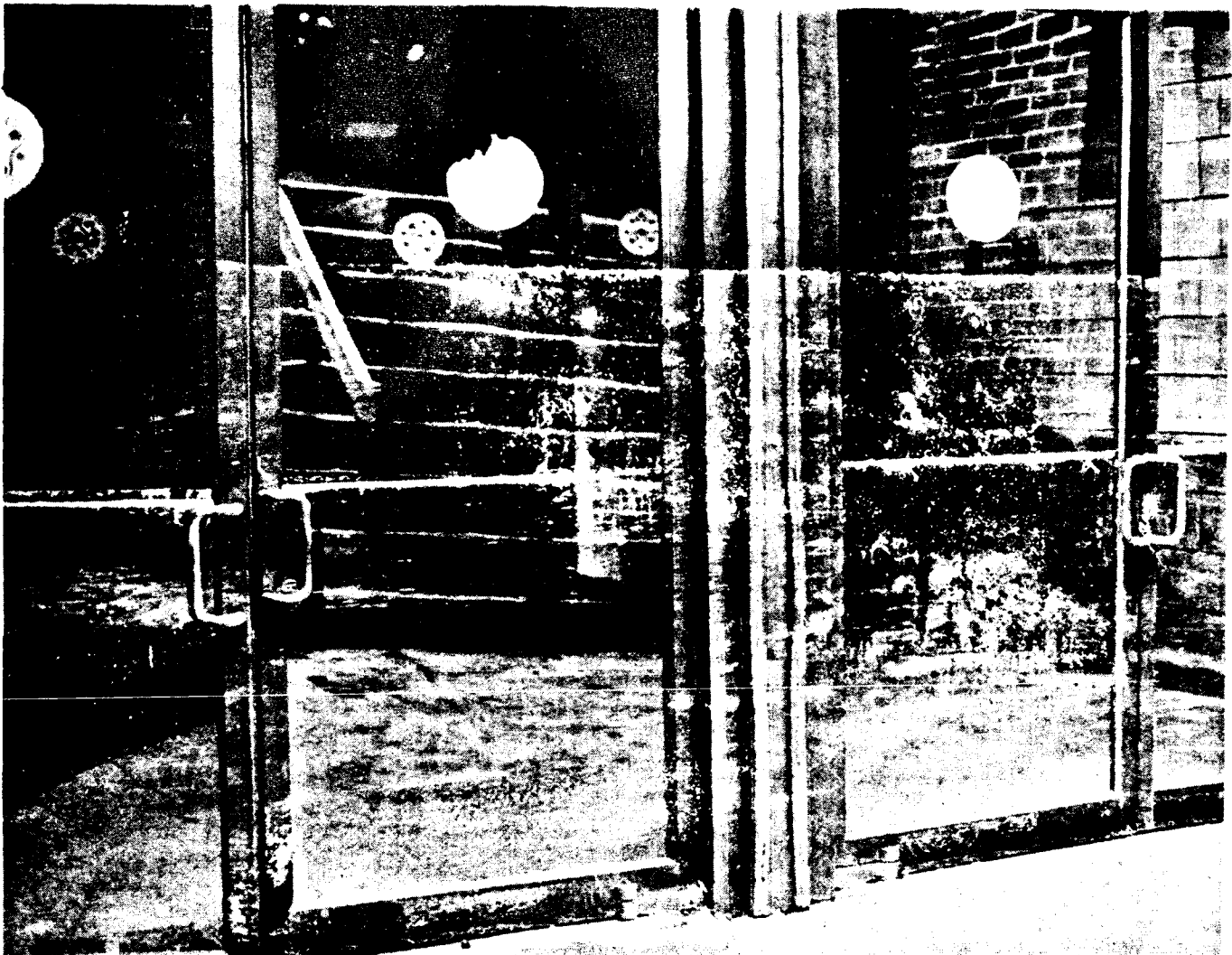
GRADUATE PHYSICS BUILDING DOOR is marked with mud at the four-foot high water mark after flooding yesterday.
