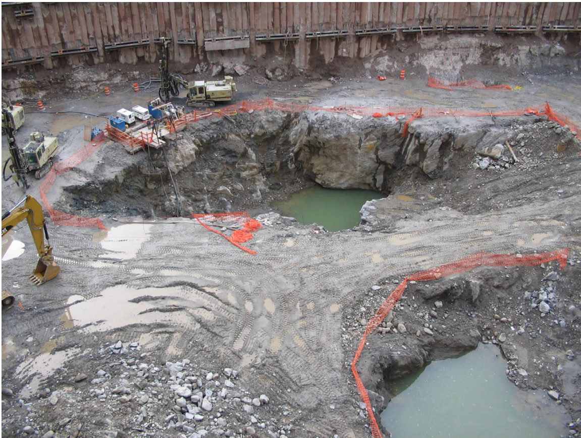
Figure 5 – Two large depressions beneath the Tower 4 site. The western basin (seen at top, facing west) had no outlet. Across the site, bedrock was initially excavated down to El. -60' and the basin bottomed out, under the green pond, at El. -100'. The pond fills a circular whirlpool and plunge pool below a near vertical cliff. During the geotechnical investigation a boring located just behind the cliff face penetrated 11' of pegmatite before entering 32' of till below. A boring on the opposite, eastern side of the basin also penetrated a small ledge of bedrock above till. The eastern depression, lower right corner, was never fully excavated so its true extent is not known. A temporary secant wall keyed into the original top of bedrock is seen along the top of the photo. (Digital image by C. J. Moss.)
