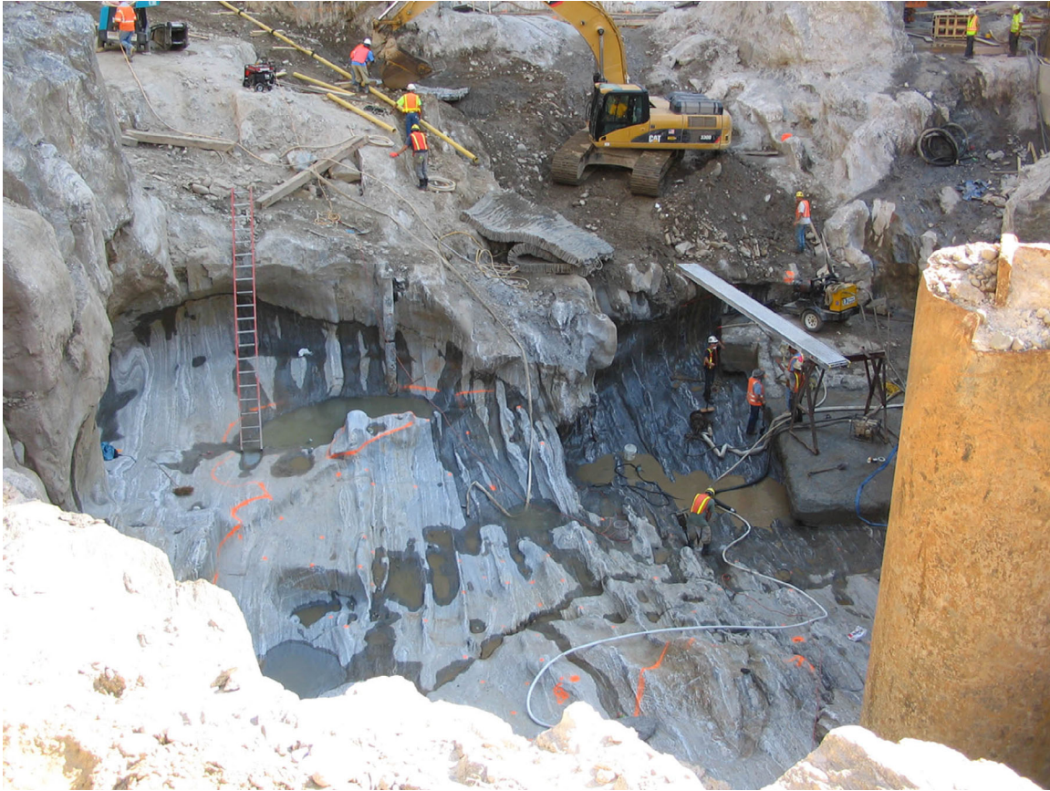
Figure 12 – “Waterslides” run down the north face of the west depression into the basins below. The more gneissic layers (white) resisted erosion and form ridges. The more micaceous schistose layers (gray) were more easily eroded and form channels. Erosion follows along the foliation. The only features that cut across the linear foliation are the round whirlpools. Overhangs create a “cave” like structure around the upper basin, which has higher ground in the center as swirling sediment scoured down the edges. A mid-level basin is in the center, and the lower basin that bottomed out at El. -100’ is center right with a slab of mass fill concrete already poured. (Digital image by C. J. Moss.)
