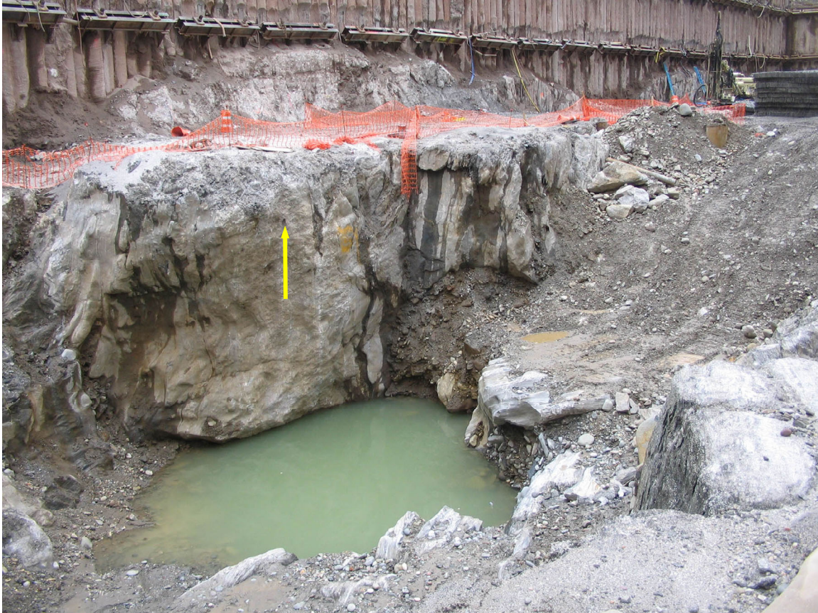
Figure 7 – Northwestern face of the west depression. At top, temporary secant wall sits above the original top of bedrock surface. Densely packed, bouldery till is seen in the center, filling a large void under the cliff face that was scoured by a plunge pool. Center right is a large, flat slab of polished, native bedrock that was originally thought to be a rock ledge until the underlying till was removed. Potholes, some still filled with till, are scattered along the sides. Green pond fills the lowest level whirlpool. Yellow arrow points to boring that cut through the upper ledge. (Digital image by C. J. Moss.)
