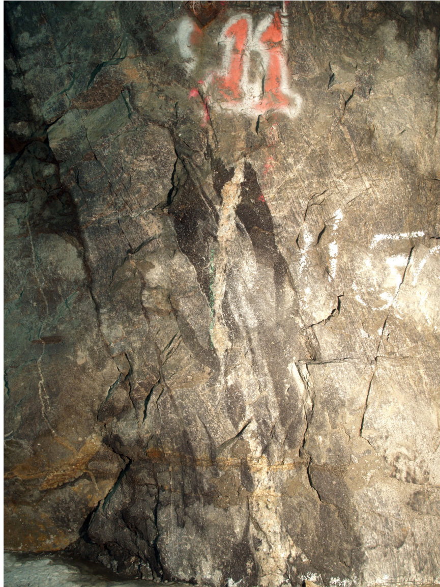
Figure 9 - Diffuse xenoliths of Fordham mafic gneiss flattened into foliation of Yonkers Gneiss near contact zone. Note late pegmatite dike cutting across the xenolith-Yonkers boundaries. Station 5+65, north wall raw water tunnel, Croton Water Treatment Plant, Bronx, New York (Digital image by C. Merguerian).
