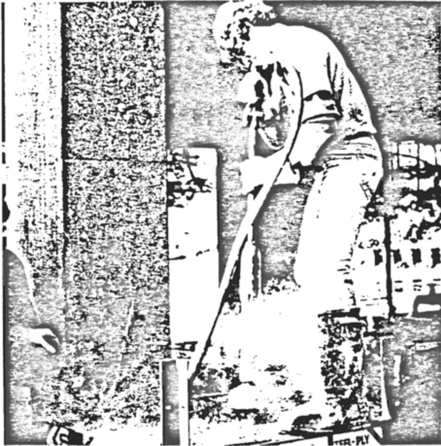
Figure VIII-1. Compacting a 1 yd 3 block.
