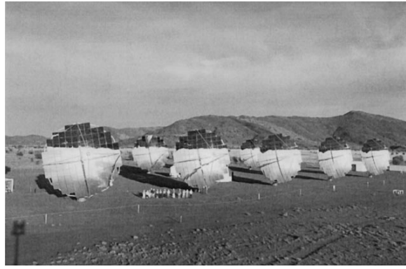
Fig. 2. To dramatize the impact of the new high-efficiency III–V solar cells on solar concentrator technology, each of these nominal 20-kW dish concentrators developed by Solar Systems Pty Ltd in Australia could be rated at over 30 kW simply by replacing the crystalline silicon solar cells with III–V cells in each receiver of the sun’s rays.
