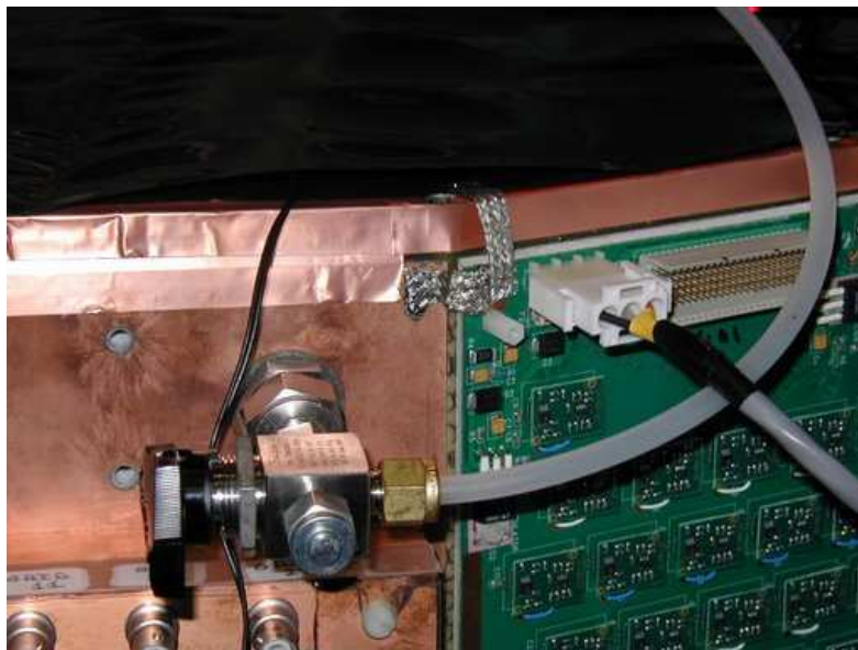
Figs. 42-44: Installing preamplifier circuit boards, one of the first preamplifier shields, grounding braids to improve noise characteristics.
