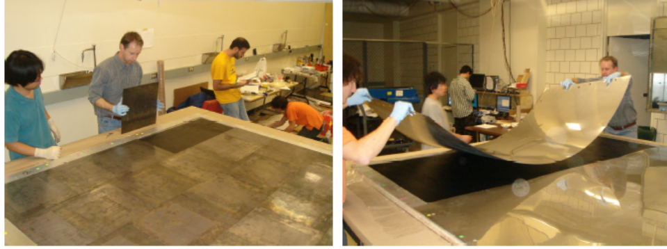
Figure 3.3: Left: Lead plates being placed into position. Right: Stainless steel sheets provide support.
