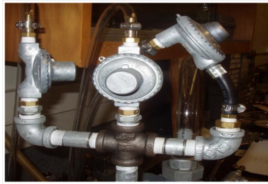
Fig. 2-2 – Natural gas pressure regulator
