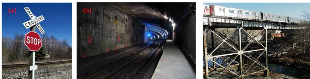
Figure 1.1 (a) No warning lights and gates in remote area, (b) subway tunnels requires significant expenditure for power wiring and (c) improper track structure monitoring and positive train control.
