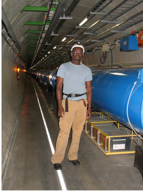
Figure 1.3: LHC dipoles (blue cylindrical tubes) in the tunnel.
