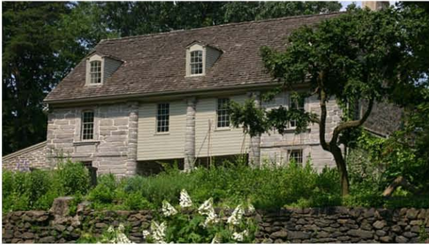
Fig. 10: View of the Bartram house (originally completed 1731, expanded between 1740–70), Bartram's Garden, Philadelphia, PA.
