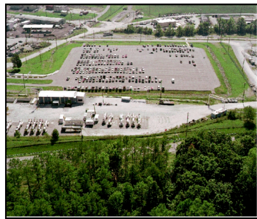
(b) transformed parking lot
