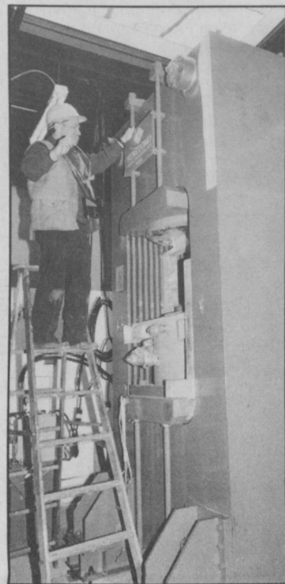
2. Dr. Robert C. Liebermann , wearing safety helmet, checks removal of safety wrappings around the press's gauges.
