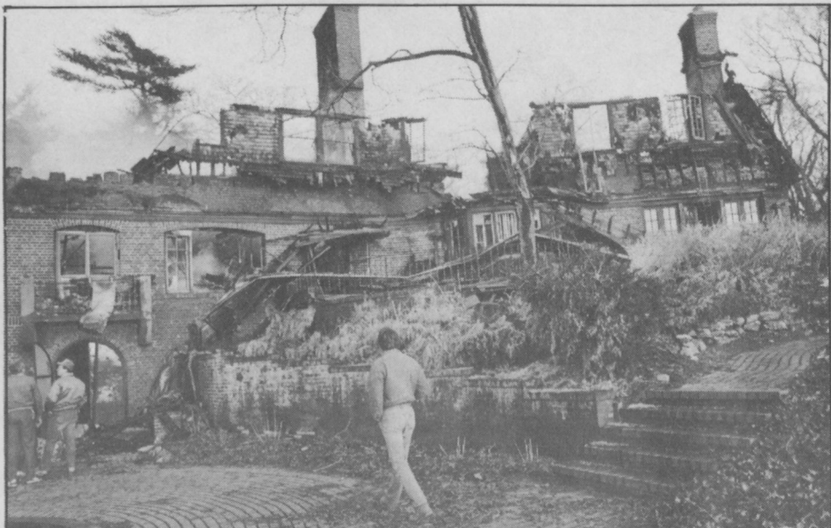
Sunwood after the fire.
