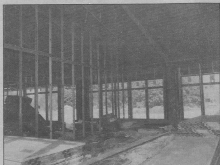
Construction on the Long Island State Veterans Home.
