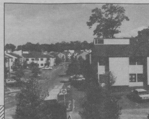
Chapin Apartments have undergone an internal and external facelift over the past two years.
