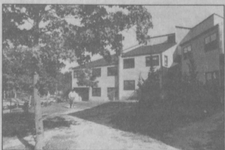
The Chapin Apartments are experiencing a massive interior and exterior reconstruction program that will be completed by next June.
