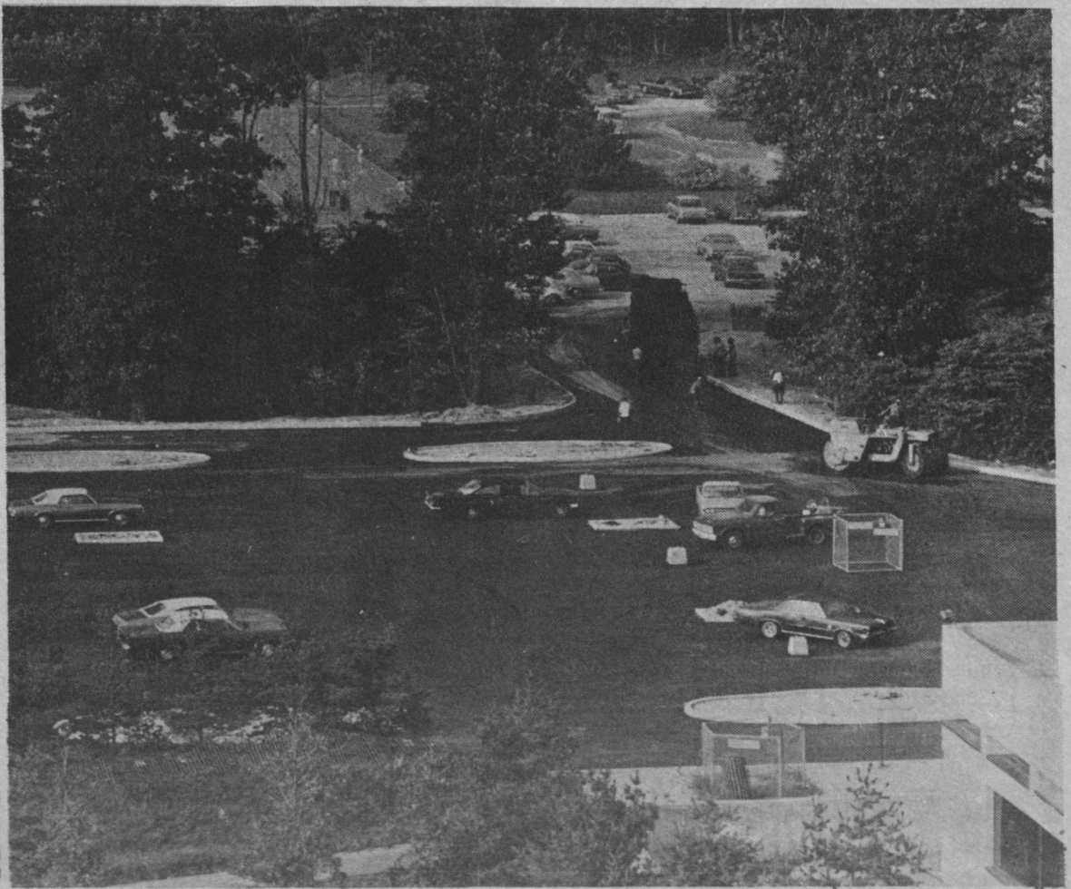
Work continued last month on repaving the Union-Infirmary parking lot.
