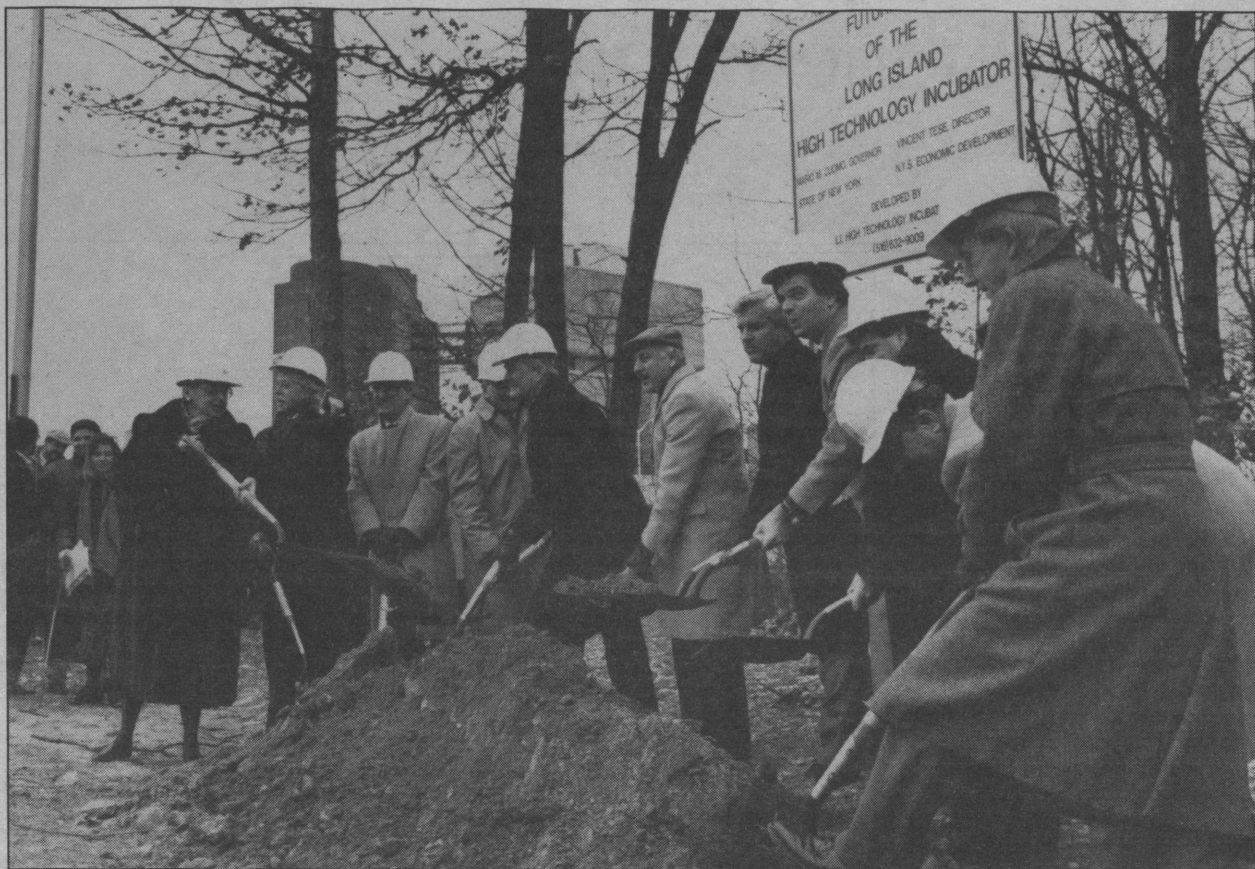
Shovels raised, academic, governmental and business leaders dig into the cold ground at the site of the Long Island High Technology Incubator when ground was broken for construction in January.
