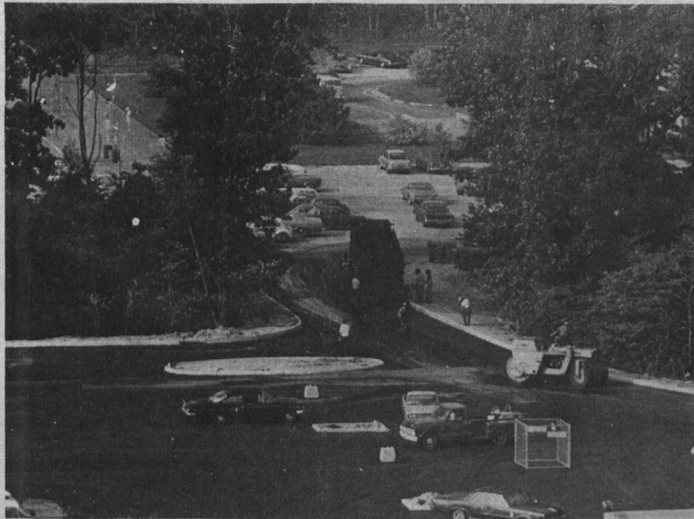
STONY BROOK UNION Parking Lot nears completion.
