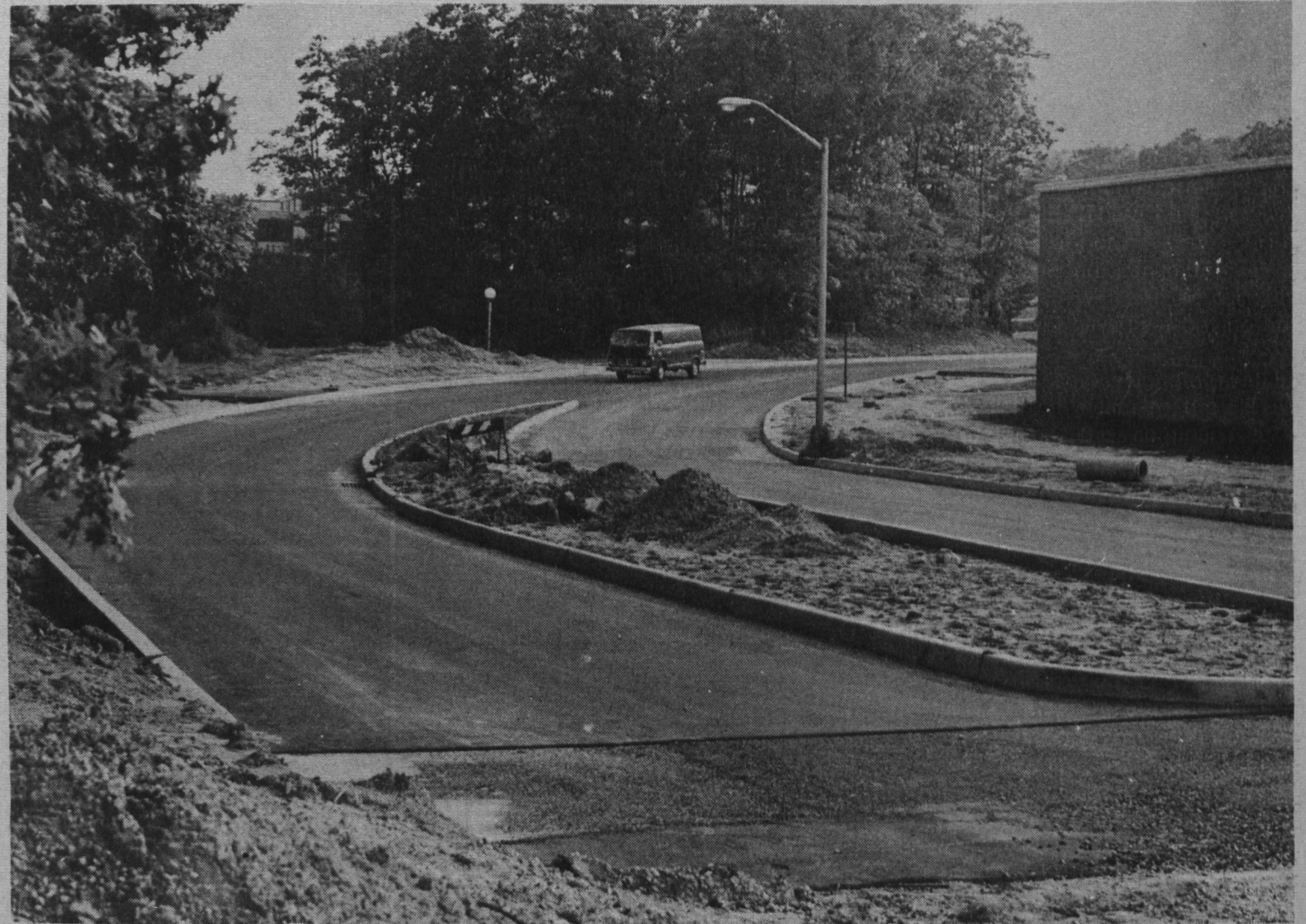
Biology Service Road, which had been closed to allow workmen to widen and repave it, has since been reopened.
