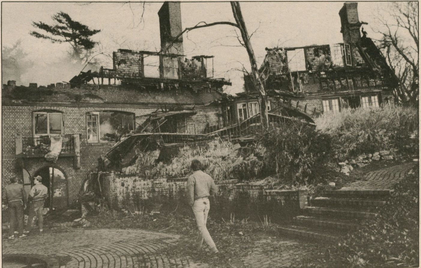
Sunwood after the fire.
