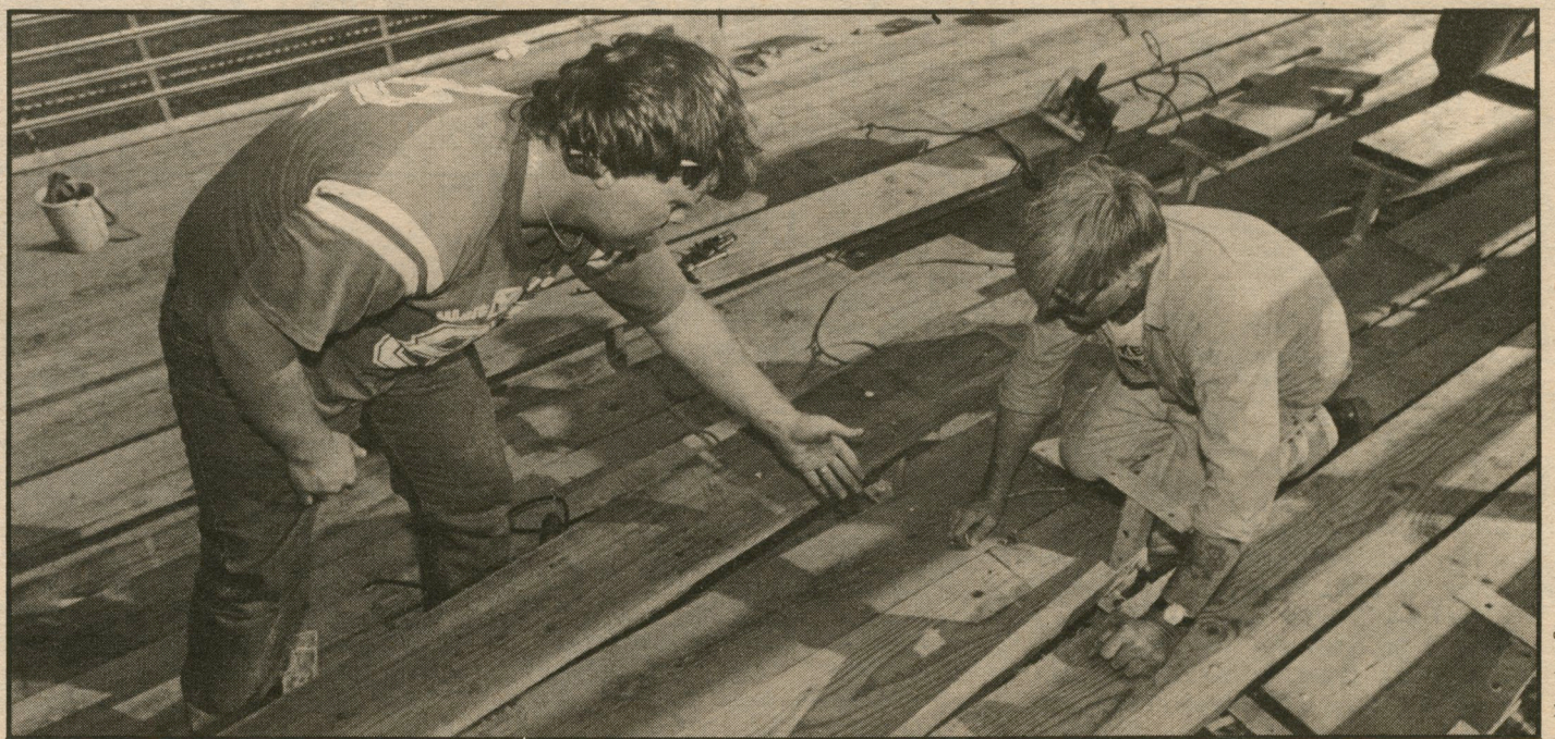
Workers complete construction of football-lacrosse bleachers seating 1,500.
