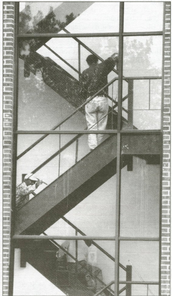
Workmen repair staircases in the Administration Building parking garage
