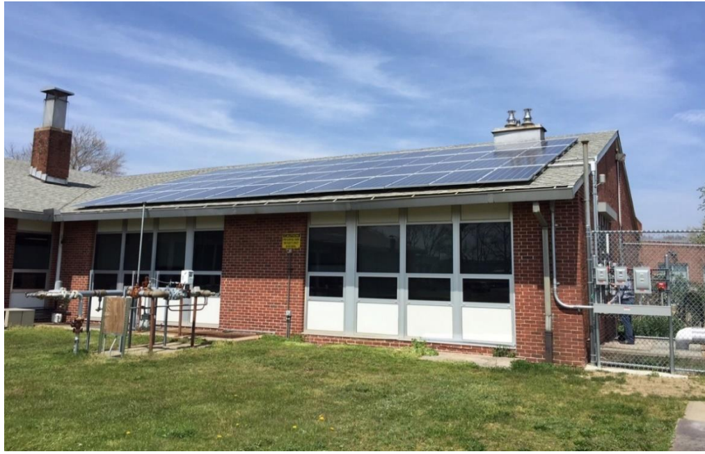
Figure 8. PV system installed for the project, on the roof of one of the Suffolk County buildings powering LED based lighting system located in Yaphank, NY
