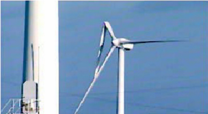
Figure 1.4 An example of blade damage
