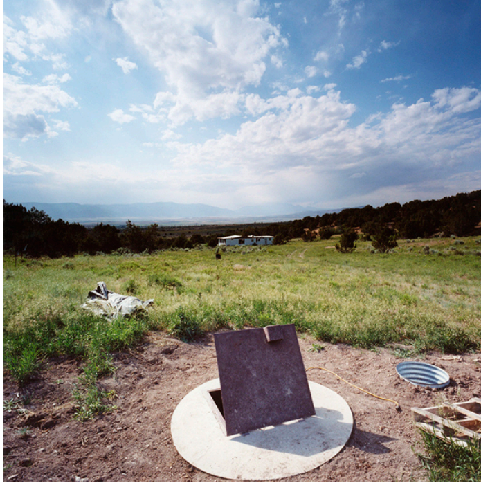
Figure 7: Entrance and air vent for a group shelter in Montana. 27
