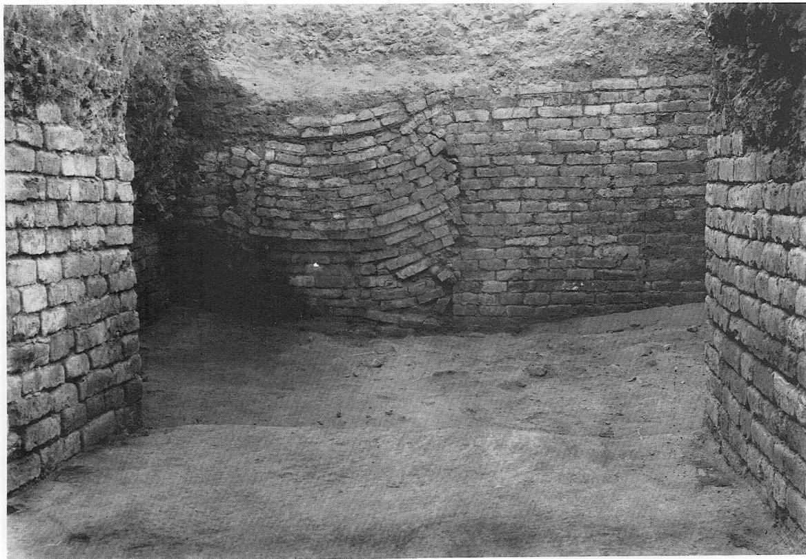
(b) Room 7: the doorway leading to Room 11, shewing the collapsed brickwork of its blocking. (p. 12)
