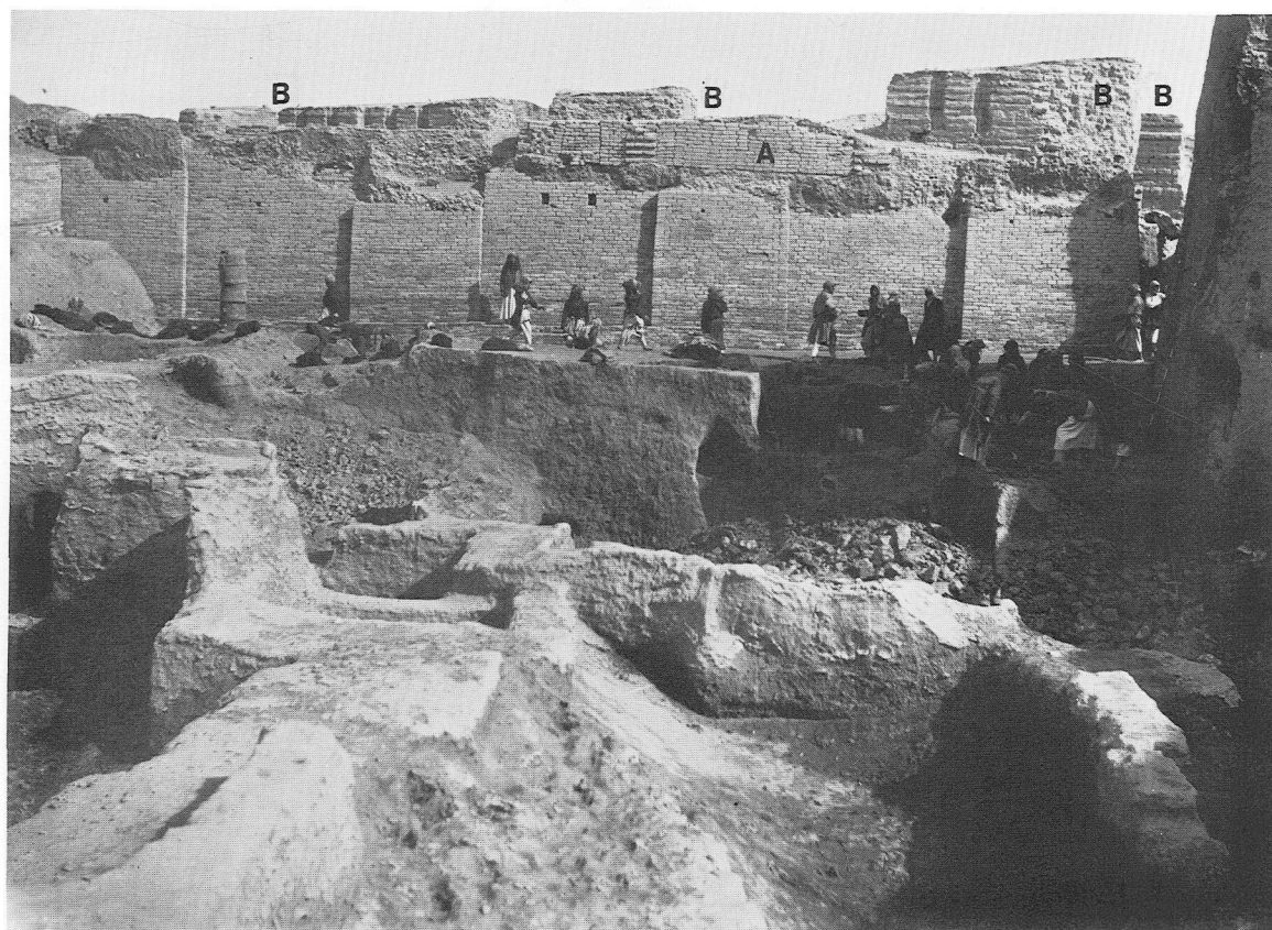
(a) The SW wall seen from the Royal Cemetery area. Above it (A) Kassite house walls; (B) Nebuchadnezzar's Temenos Wall. (p. 1)
