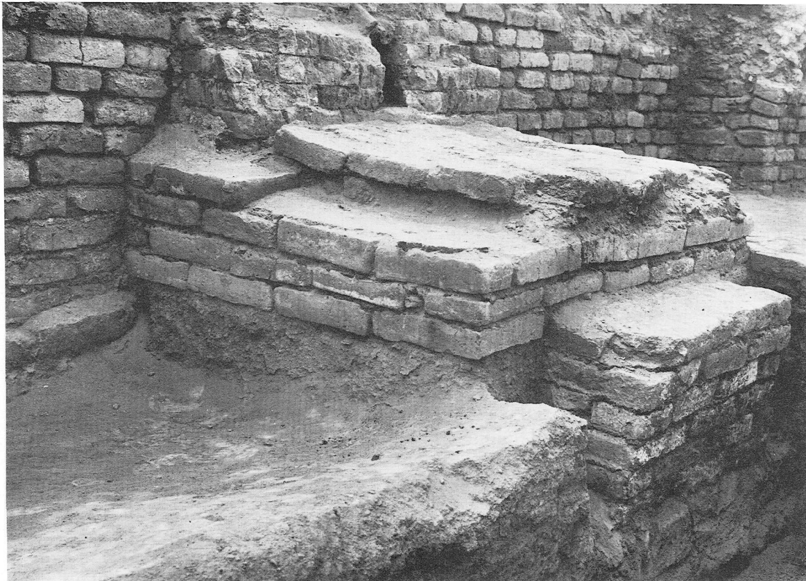
(b) Ur-Nammu's drain in the NE wall: the lower part of the vertical shaft and the outlet. (pp. 46, 48)
