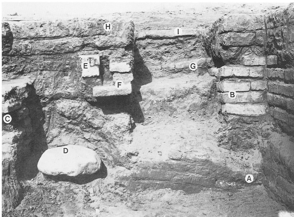
(b) Room 14 (p. 52) shewing A, the mud-brick wall of Ur-Nammu; E, F, support and base of door frame; B, Larsa period burnt-brick wall; G, threshold; C, remains of hinge-box; H, Neo-Babylonian mud-brick step; D, socket-stone; I, pavement of Nebuchadnezzar.
