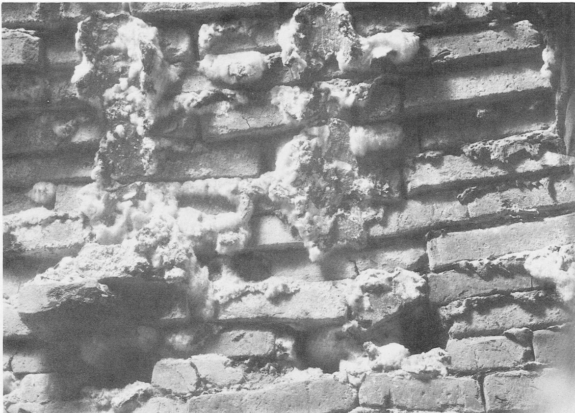
(b) Tomb-chamber 3: detail of the corbelled roof showing on the brickwork the bitumen coating of the centering-beams (the grain of the wood is visible). (pp. 18, 35)
