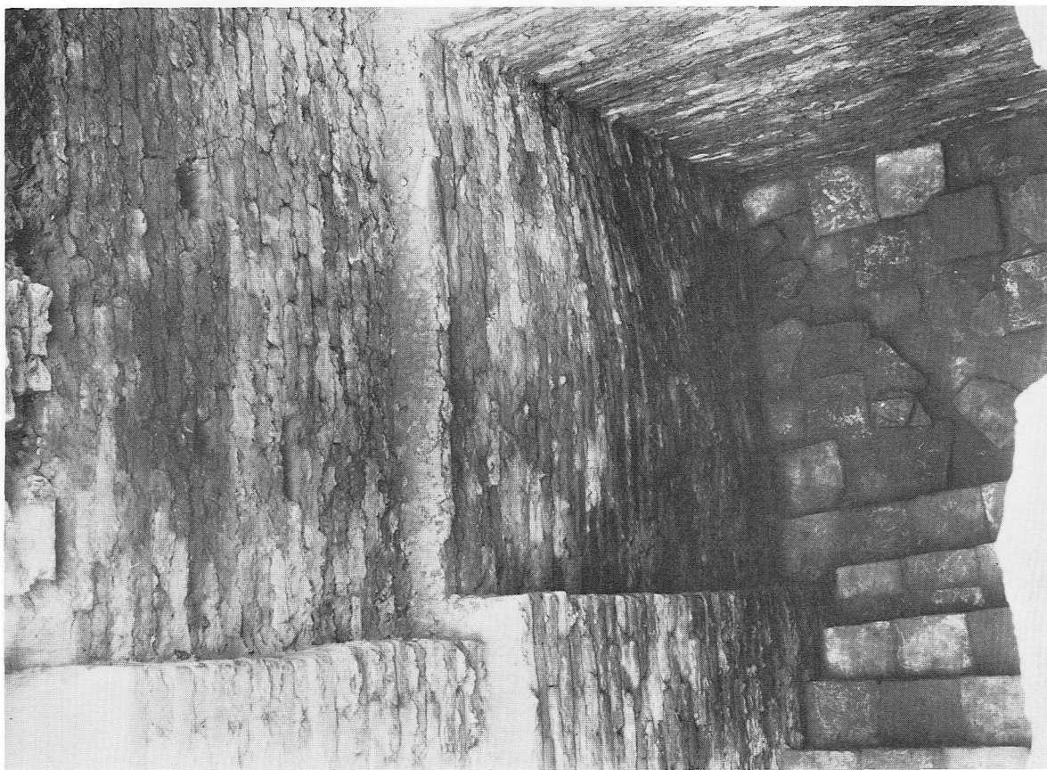
(a) The blocked entrance to the SE tomb chamber. (p. 28)
