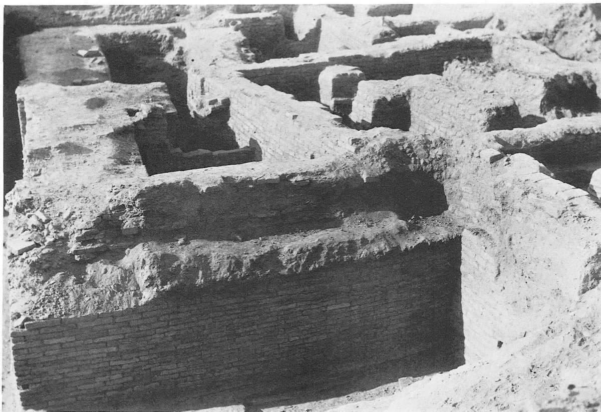
(a) General view of the building from the SE. (p. 30)
