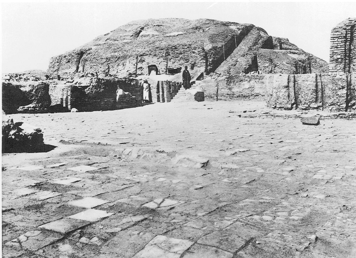
a. View across courtyard of E-dub-lal-mah showing the steps to the Ziggurat terrace and the gateway of the continuation of the Via Sacra .
