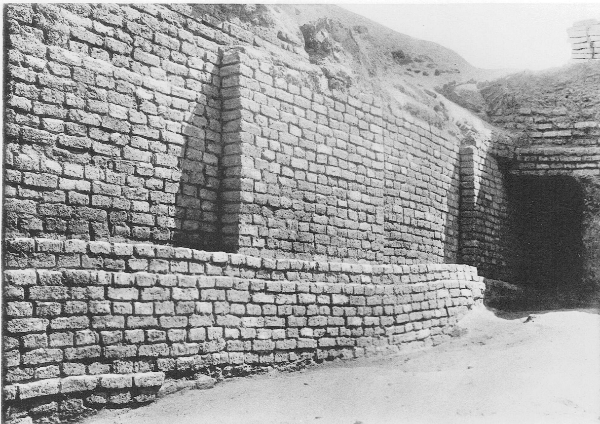
a. The outer face of the butressed wall dividing sections B and C.
