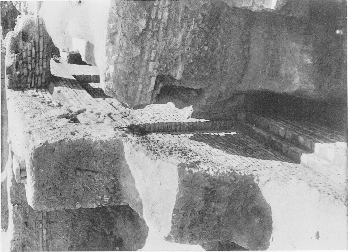
b. View looking SE along the outer (SW) wall of the B range.
