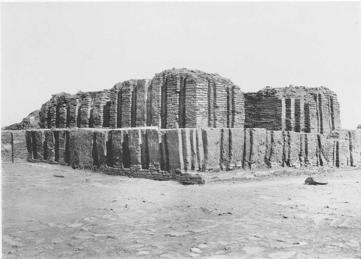
b. General view from the South, after final clearing
