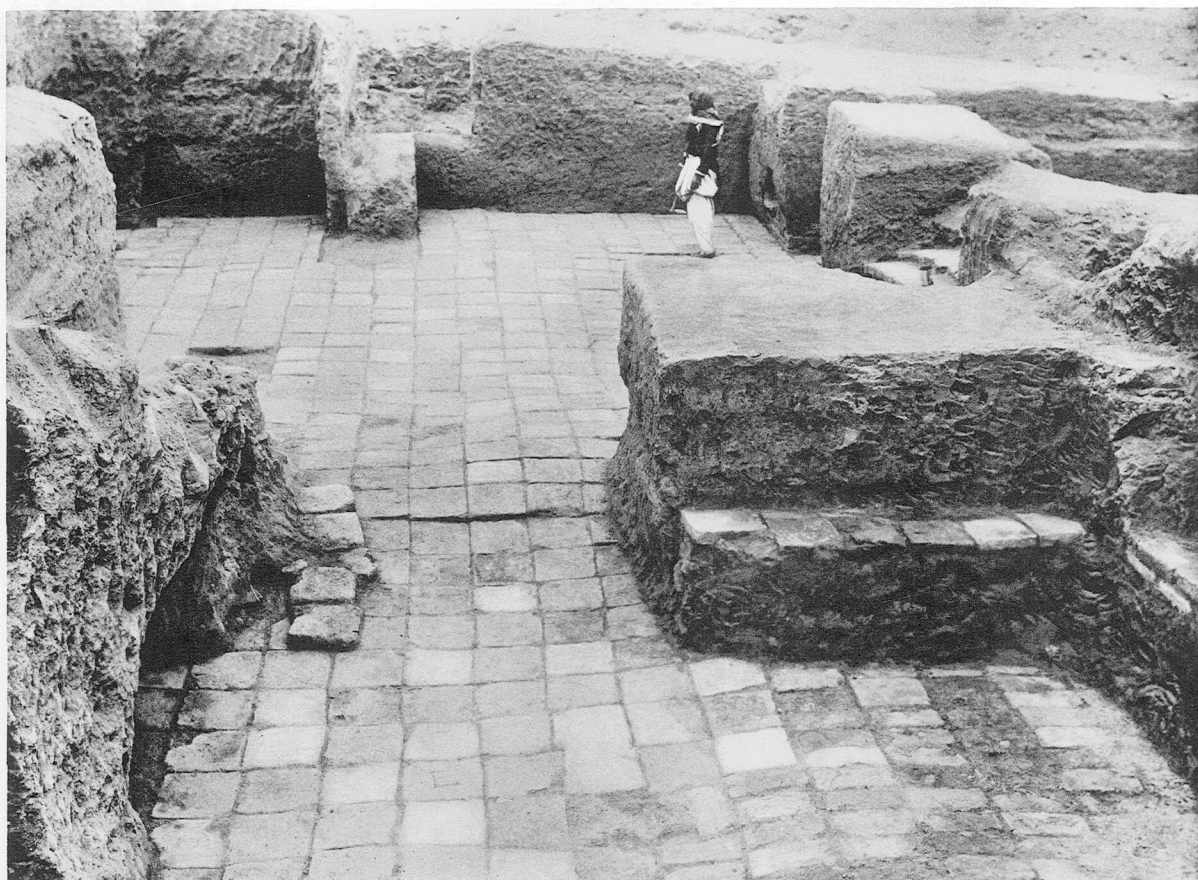
a. Level 2 ; Room 2 in course of excavation. The pavement is that of level 2, the walls are those of Nebuchadnezzar's corner fort ; against the near wall on the right is a strip of the Level 2 bis pavement.
