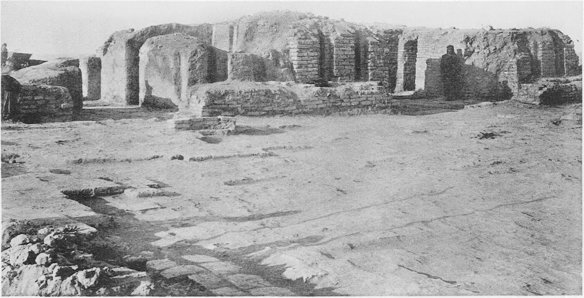
(a) General view from the South
