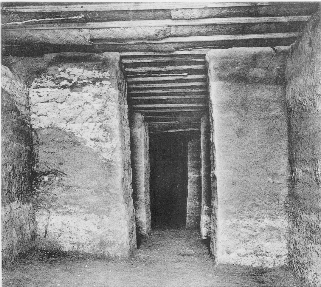
(b) The entrance passage after roofing; looking south-east
