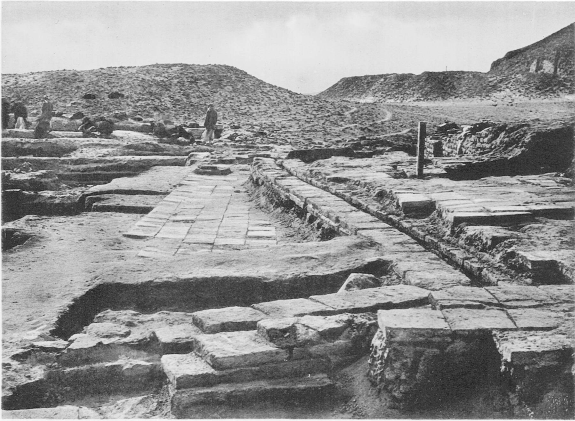
(a) Room 1. The Persian pavement and drain in front of the shrine ; below it, the Nebuchadnezzar pavement
