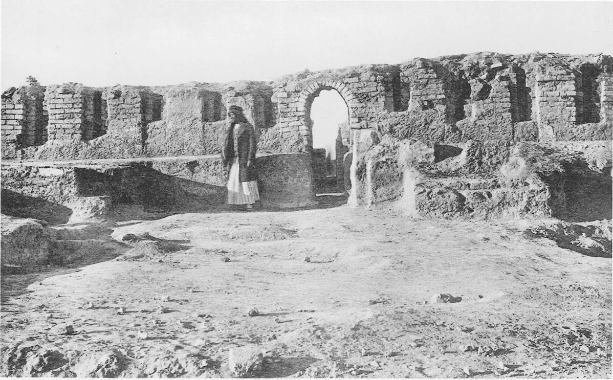
(a) General view from the South-West (some of the late walls removed)
