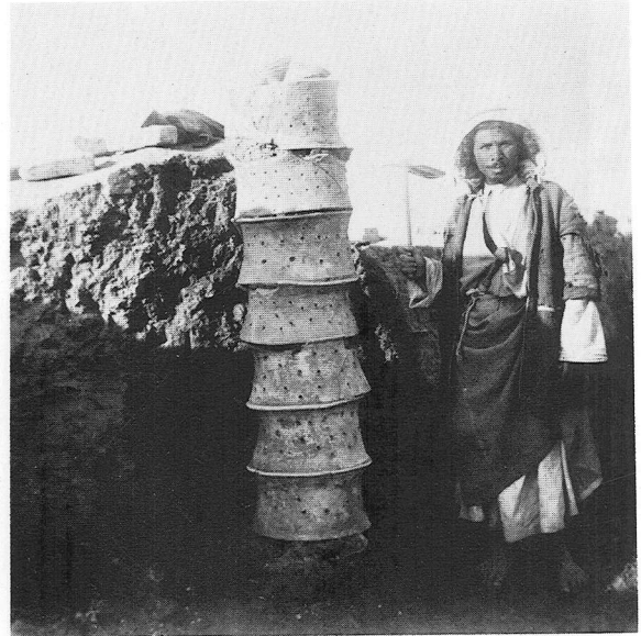
b. A typical Larsa drain (EH site)
