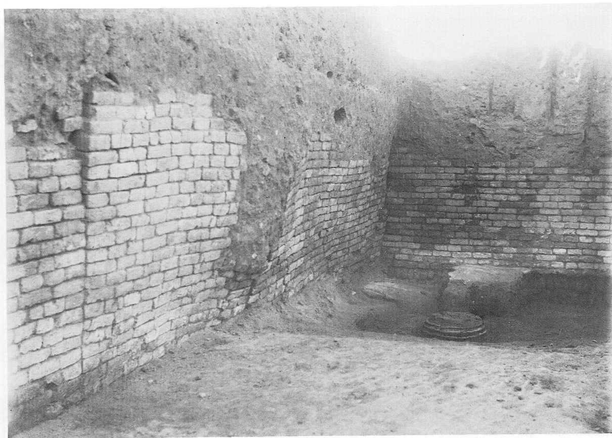
b. Room C30, the west corner
