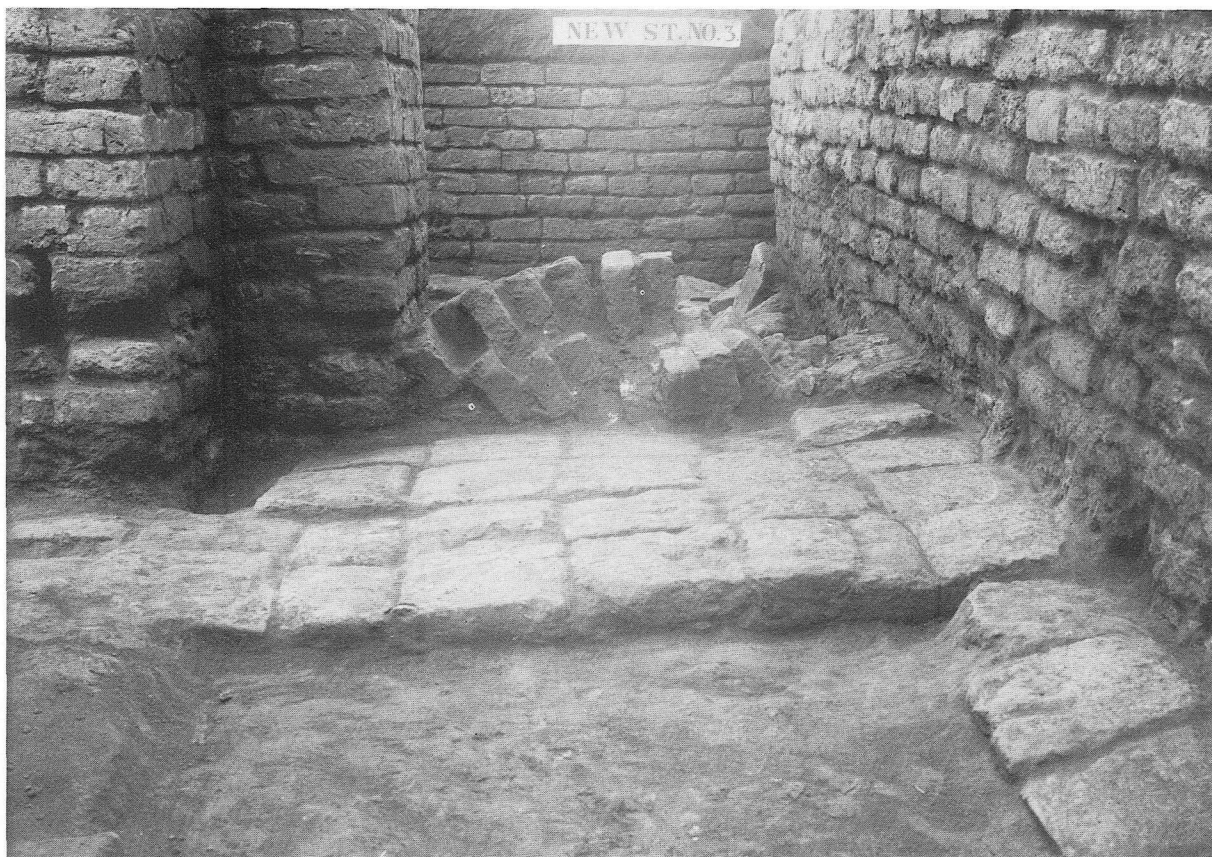
a. No. 3 New Street. The doorway of the domestic chapel (Room 6) with the fallen brick arch in situ
