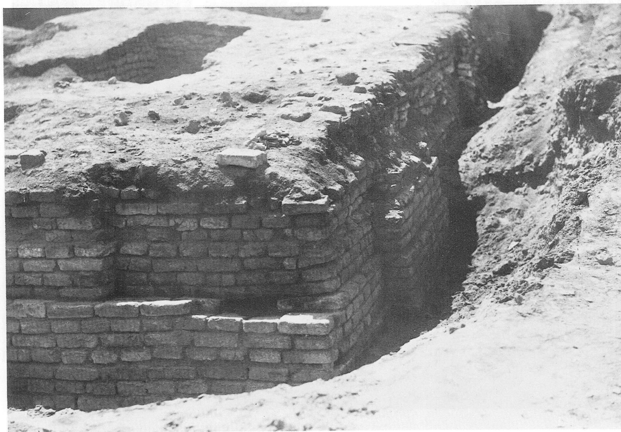
b. The Enki Temple of Rim-Sin; the stepped foundations of the outer wall, west corner THE TEMPLE OF NIN-GIZ-ZIDA AND OF NIN-EZEN and THE ENKI TEMPLE
