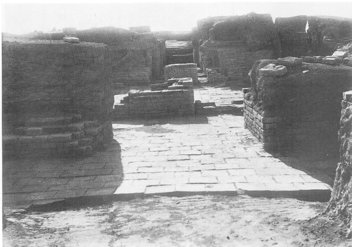
b. View from C3 through C7 to the sanctuary, showing the Hammurapi base and, behind it, the brick altar
