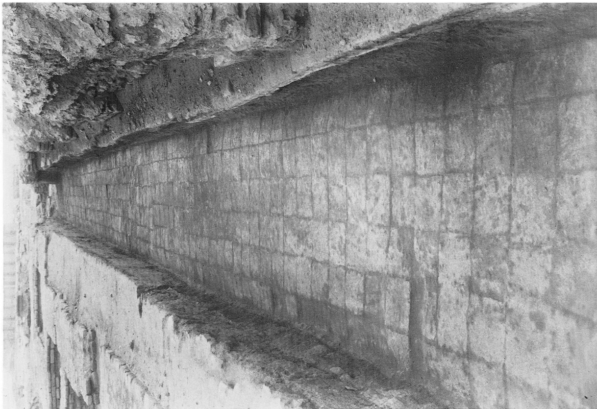
b. The long passage on the NW side, with paving by Amar-Suena
