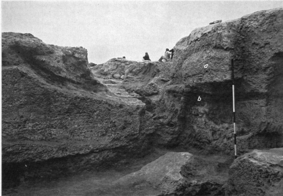
FIG. 65.—PART OF THE WEST WALL OF SIN TEMPLE X, SHOWING A BUTTRESS (a) ABOVE AN ASH LAYER (b) WHICH COVERED THE DEBRIS OF EARLIER PRIVATE HOUSES
