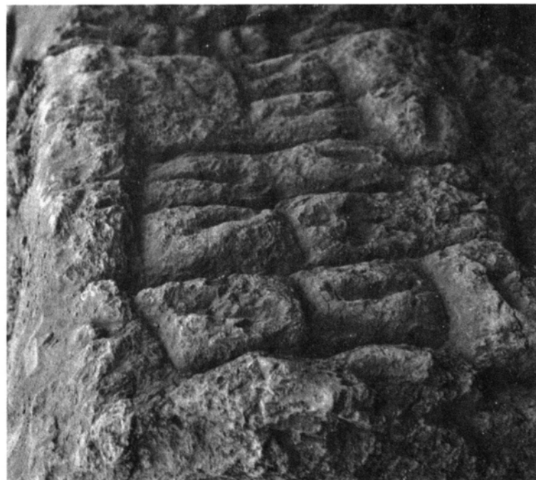
FIG. 147.—PLANO-CONVEX BRICKS USED IN THE SQUARE TEMPLE
