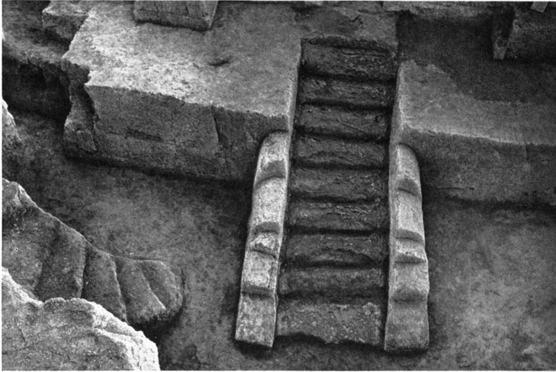
FIG. 40.—STAIRWAY, TERRACE, AND BUTRESSES AT THE ENTRANCE OF THE FIRST OCCUPATION LEVEL OF SIN TEMPLE VII, SEEN FROM EAST
