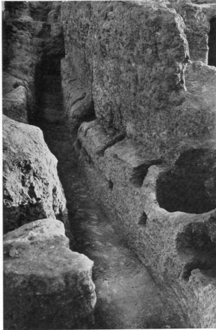
FIG. 51.—TWO ROWS OF SQUARE HOLES IN THE FACE OF THE EAST WALL OF SIN TEMPLE VIII
