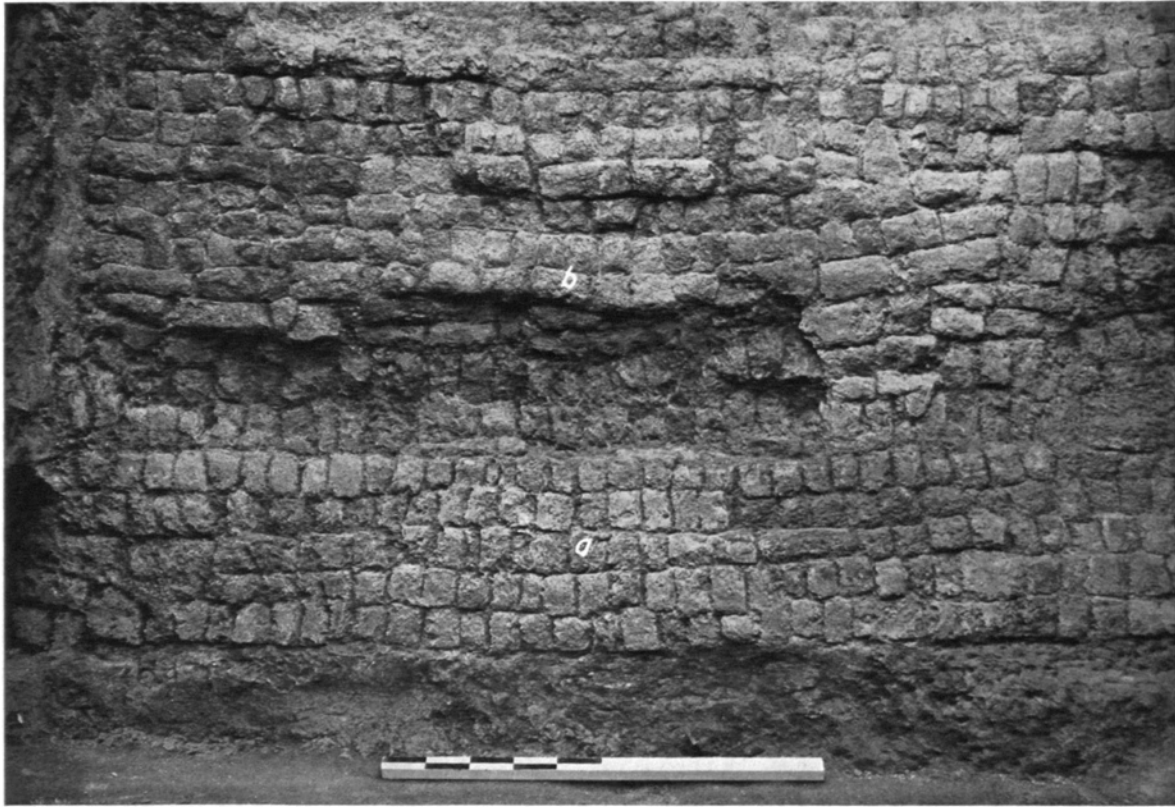
FIG. 110.—SOUTH WALL OF THE SANCTUARY, SHOWING BRICKWORK OF SIN TEMPLE III (a) AND OF THE FOUNDATIONS OF SIN TEMPLE IV (b)
