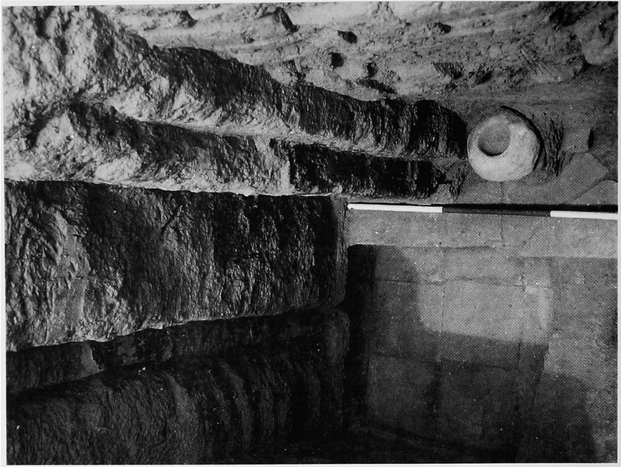
b) Great Temple: succession of Level 3 pavements, the latest represented by the door socket
