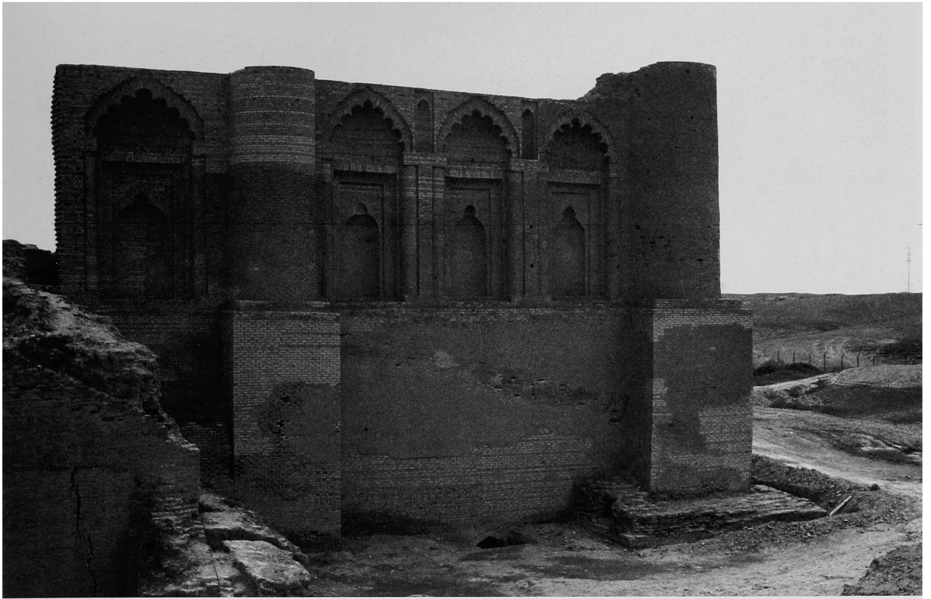
Pl. 87. Al-'Āshiq, northwest façade.
