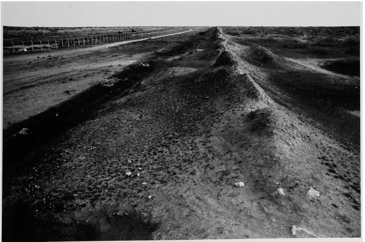
Pl. 76. Canal on the west side of the avenue in al-Mutawakkiliyya.
