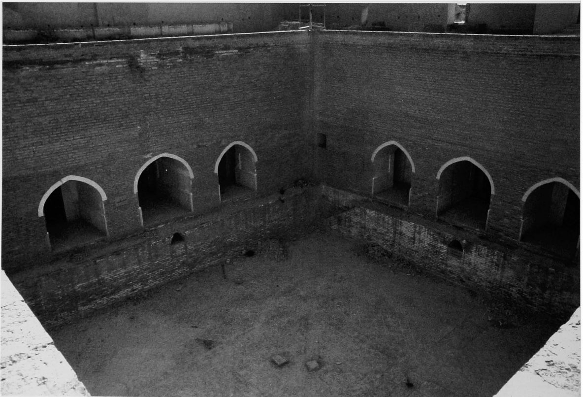
Pl. 46. The Small Serdab, view after restoration in 1987.
