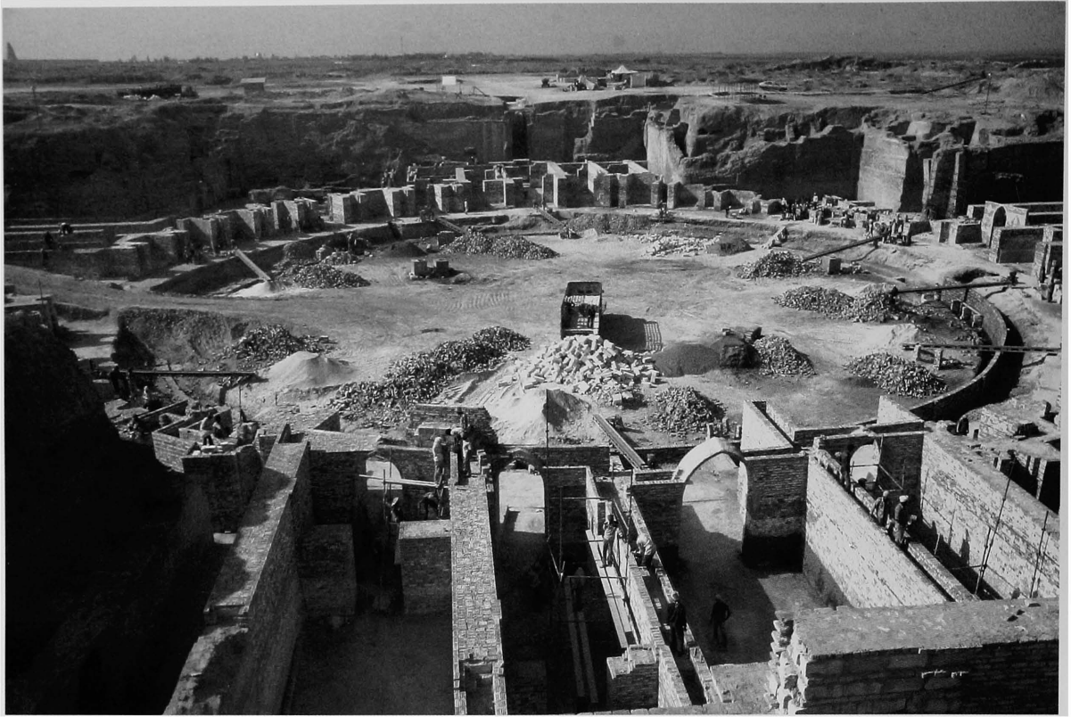
Pl. 45. The Large Serdab, view of restoration in progress in 1989.
