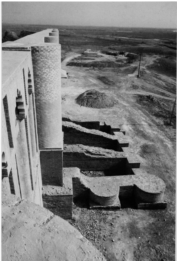
Pl. 89. Al-'Ashiq, foundation of tower pavilion.
