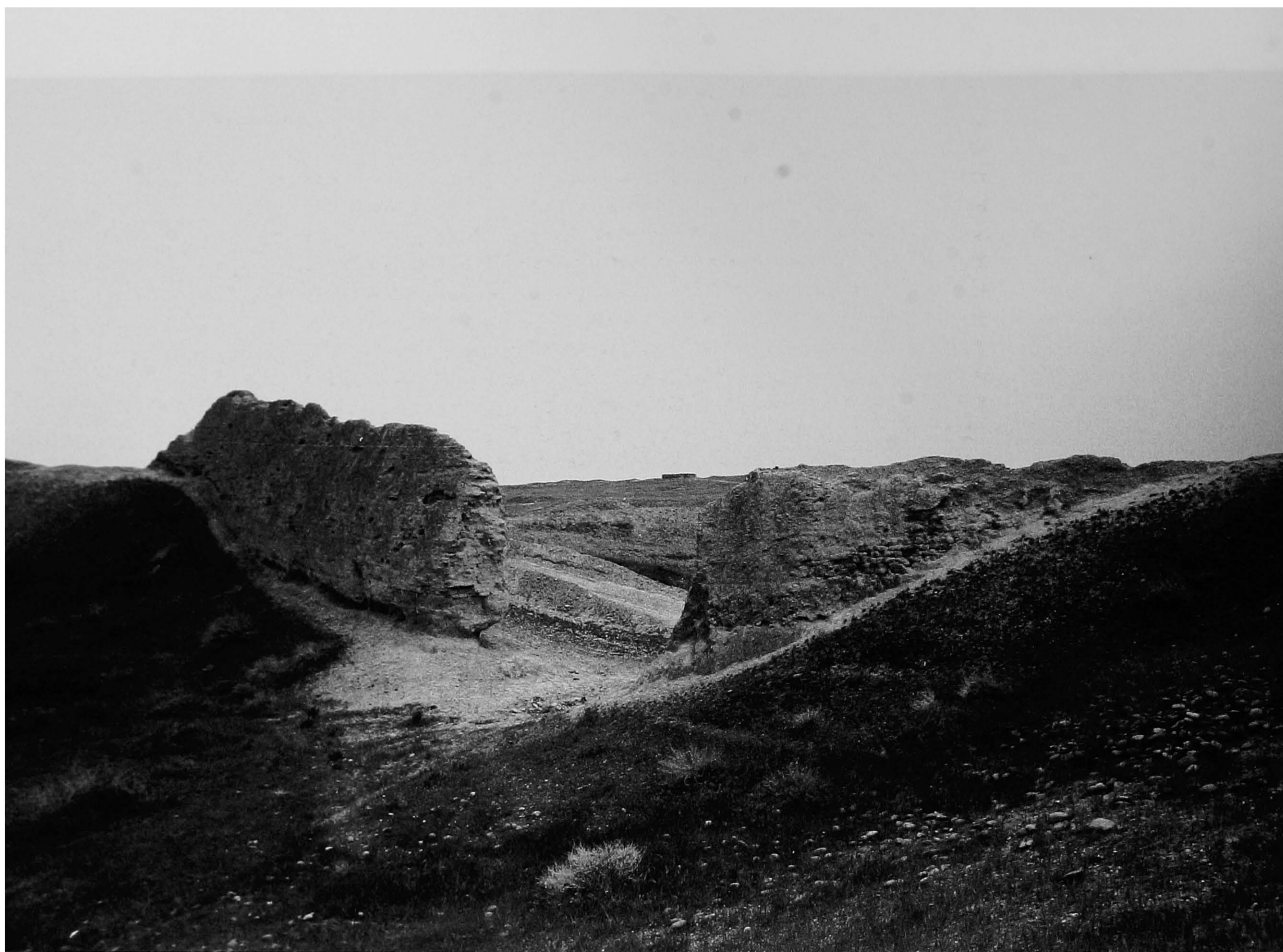
Pl. 7. The fortifications of Qal'at al-Māhūza.
