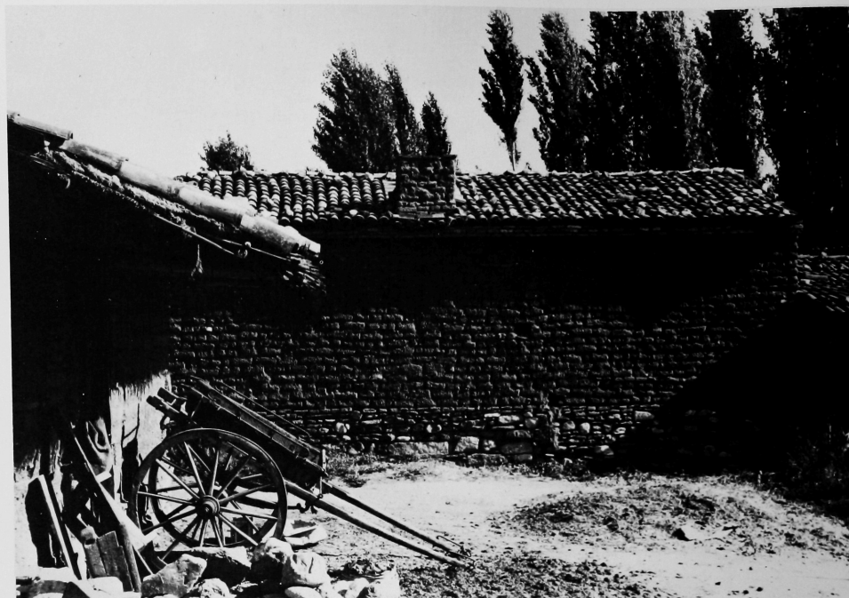
Fig. 27 Sart Mustafa, house with friezelike row of bricks under the eaves.
