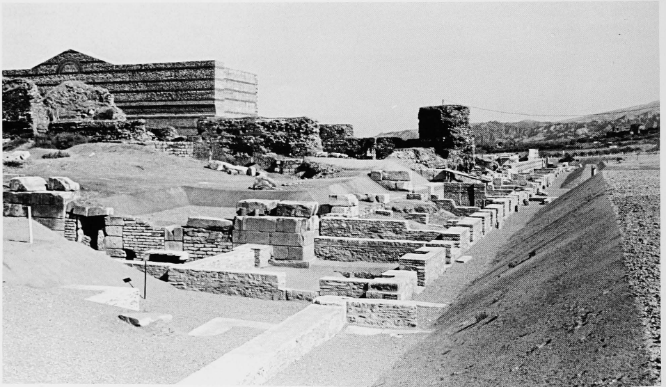
Fig. 41 The West Shops as restored, 1973. Looking NE.
