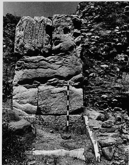
Fig. 115 Pier in NW corner with beam holes at *96.20. Top of basin shows below, 1973.
