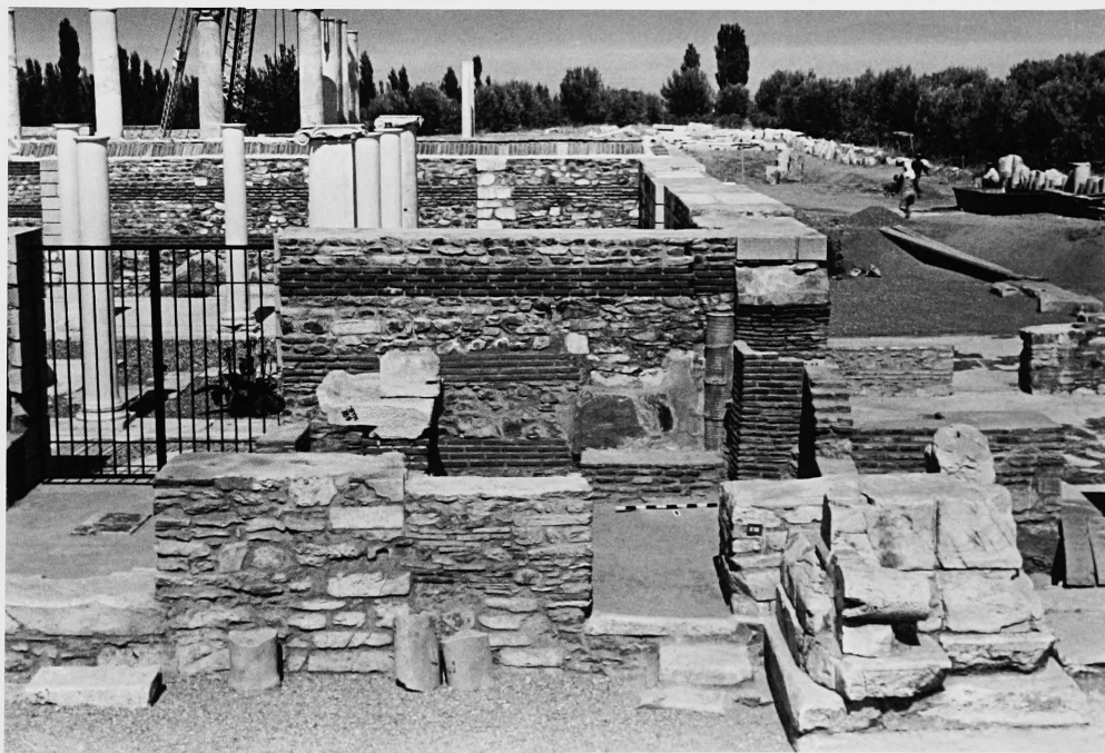
Fig. 576 E 19 as restored, 1973. Looking N.
