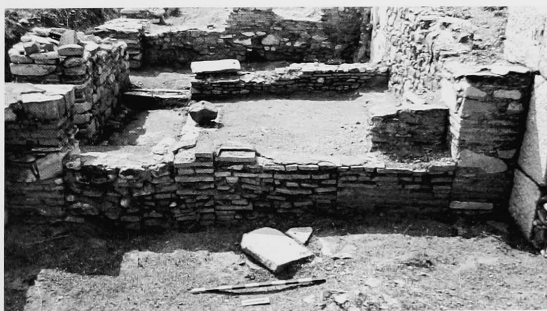
Fig. 71 Looking W into W 8 and W 9, 1969. E face of W wall of W 7 in the foreground.
