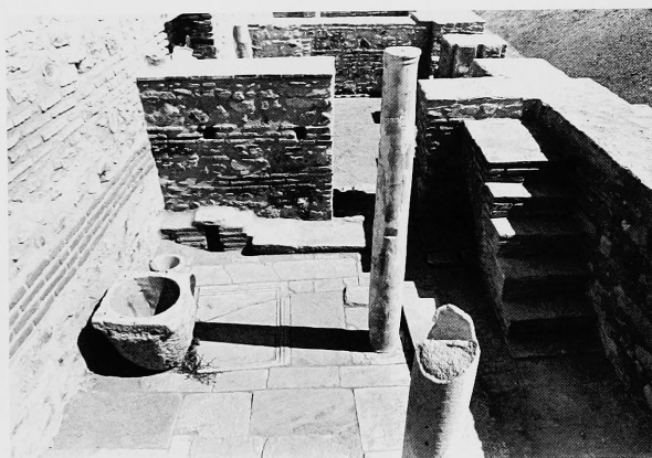
Fig. 271 E 6 looking E into E 7, as restored, 1973. The large mortar or vat was found in E 6.
