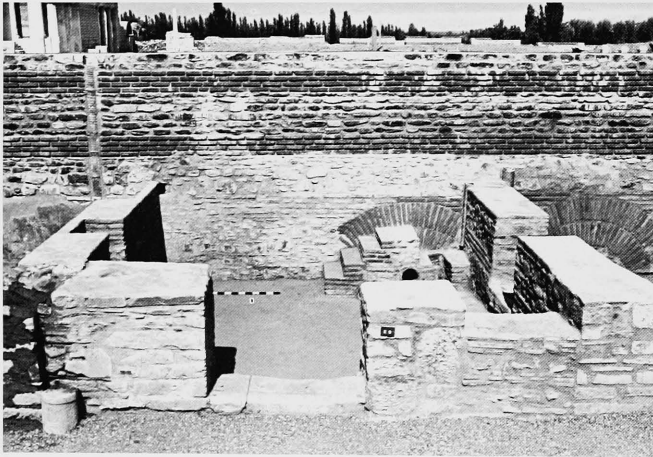
Fig. 330 E 9 as restored, 1973. Looking N.
