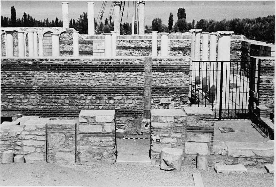
Fig. 560 E 18 and entrance to Syn Fc as restored, 1973. Looking N.
