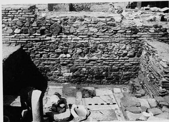
Fig. 270 E 6 as excavated, 1969. Looking N.
