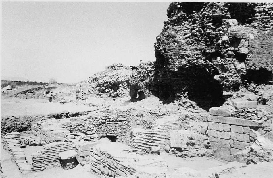
Fig. 130 W 1 (foreground) and W 2 as excavated, 1958. Looking NW.
