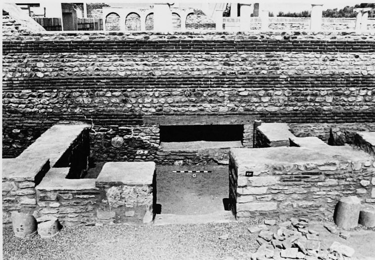
Fig. 541 E 17 as restored, 1973. Looking N.
