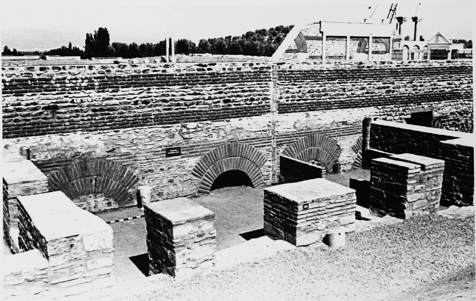
Fig. 345 E 10 and E 11 as restored, 1973. Looking NE.
