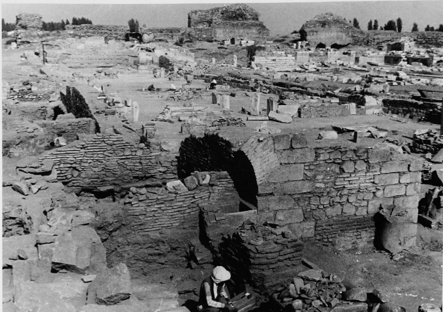
Fig. 577 The walls of E 19 abutting the S wall of the B complex, beyond the partially preserved arch. In the background, the E Shops, Syn, Pa, MC during excavation, 1963. Looking NW.
