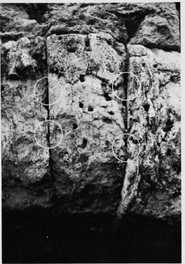
Fig. 418 SCW. Detail of wedges in keystone.
