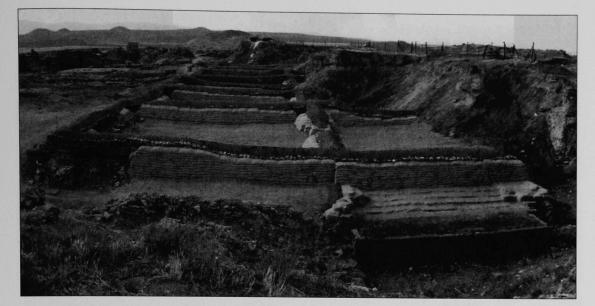
Figure 17-9 Terrace Building after interpretive stabilization. Supportive buttressing and capping protects eroded structure while providing a schematic and reversible restoration of the building plan. Pending evaluation of the stairway protection, the cinderblock encasement can be removed and the geotextile treatment extended along the steps to recover original site topography.
