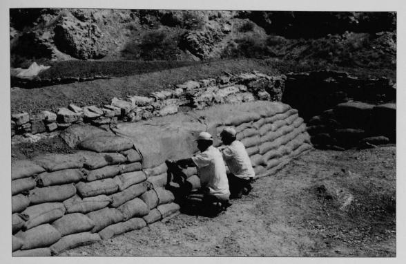
Figure 17-7 Applying protective Geotextile dressing over sandbag buttresses, August 2000.
