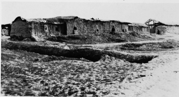
2.3. New construction on top of the defensive wall
