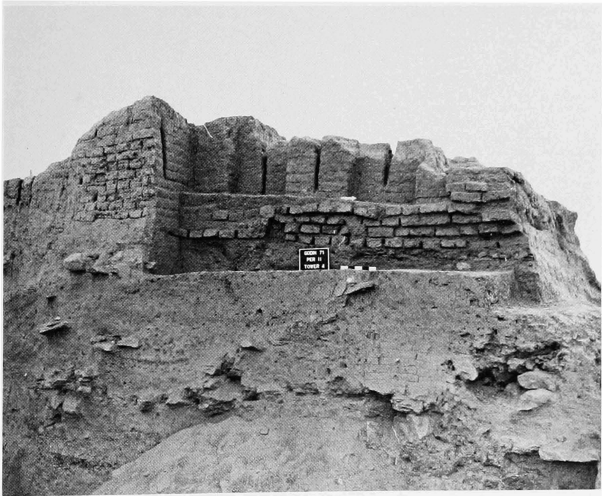
Plate XXIII: Period II, east face of tower 13 cleared back to the remaining fragment of the original fortification wall running between towers 13 and 5.
