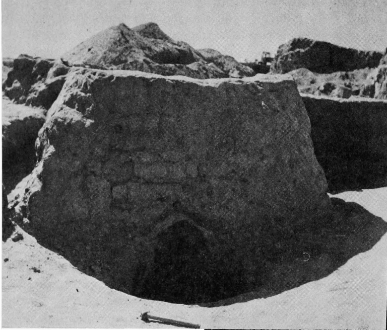
View of kiln showing opening to firebox below. Some of the plaster has been removed to show bricks.
