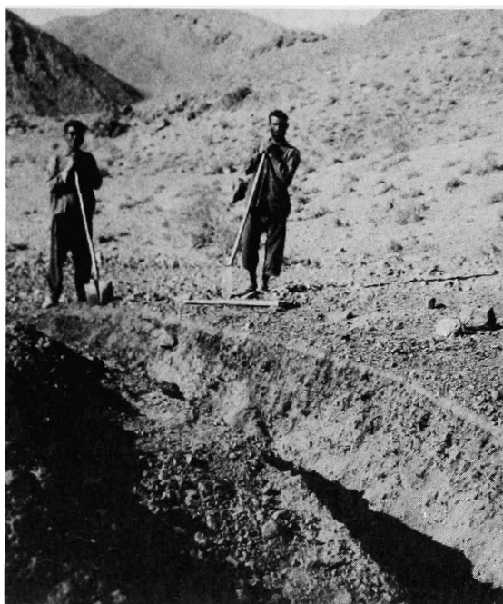
3. Our trench through cinder heap No. 1.
