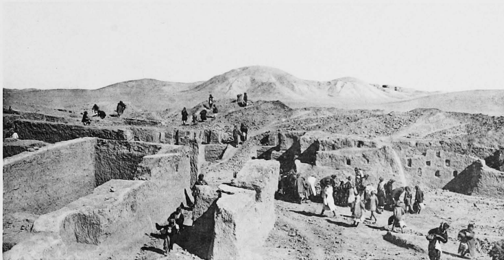
2. Excavations at the Palace later in Season.
