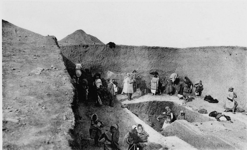
1. Wide Trench driven into Eastern Side of E-mete-ursag.
