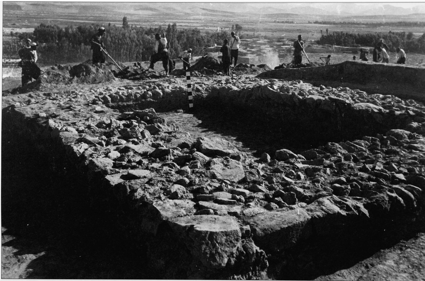
Plate G. Operation XXXIV (CC30) taken in 1960 from the northeast, showing the stone footings of Building II Phase 1.
