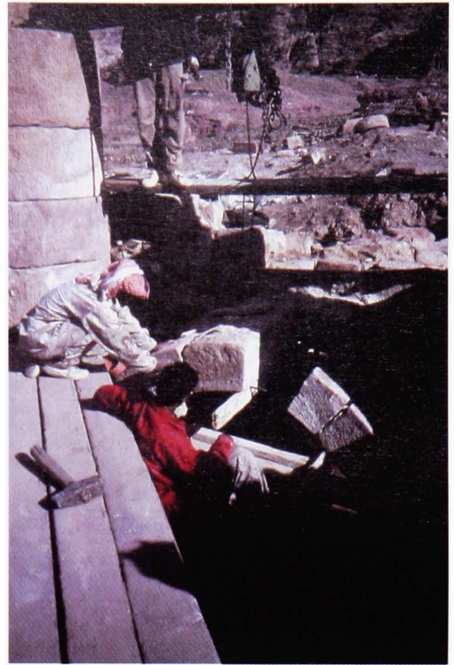
Plates 13, 14 and 15. Anastylis (reconstruction) of the Inter-columnar Wall of the West Corridor, 1997-1998.
