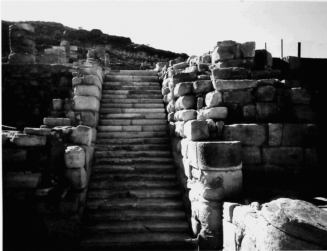
Figure 5.21. West Stairway (Laurel Stairway) after reconstruction, looking south, 1997.
