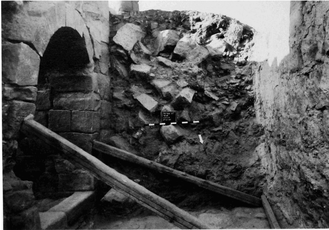
Figure 2.79. Arched doorway, West Corridor, looking southeast, 1997.
