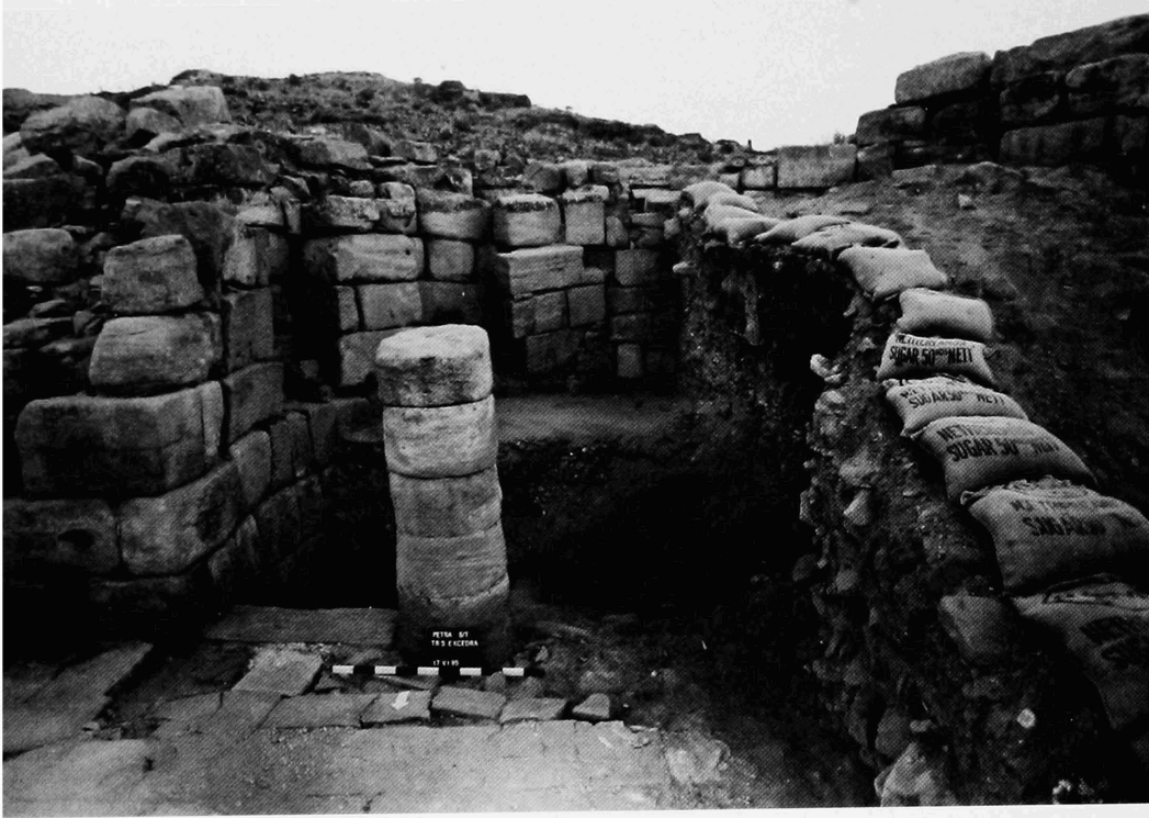
Figure 2.34. West Exedra during excavations, 1995.
