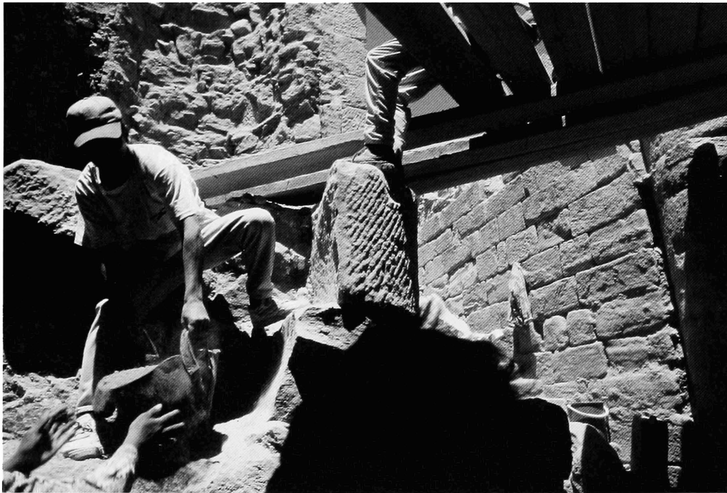
Figure 2.2. Bedouin workers removing soil from Brian Stairway and Suleiman Column, 1997. Photograph by John Forasté.
