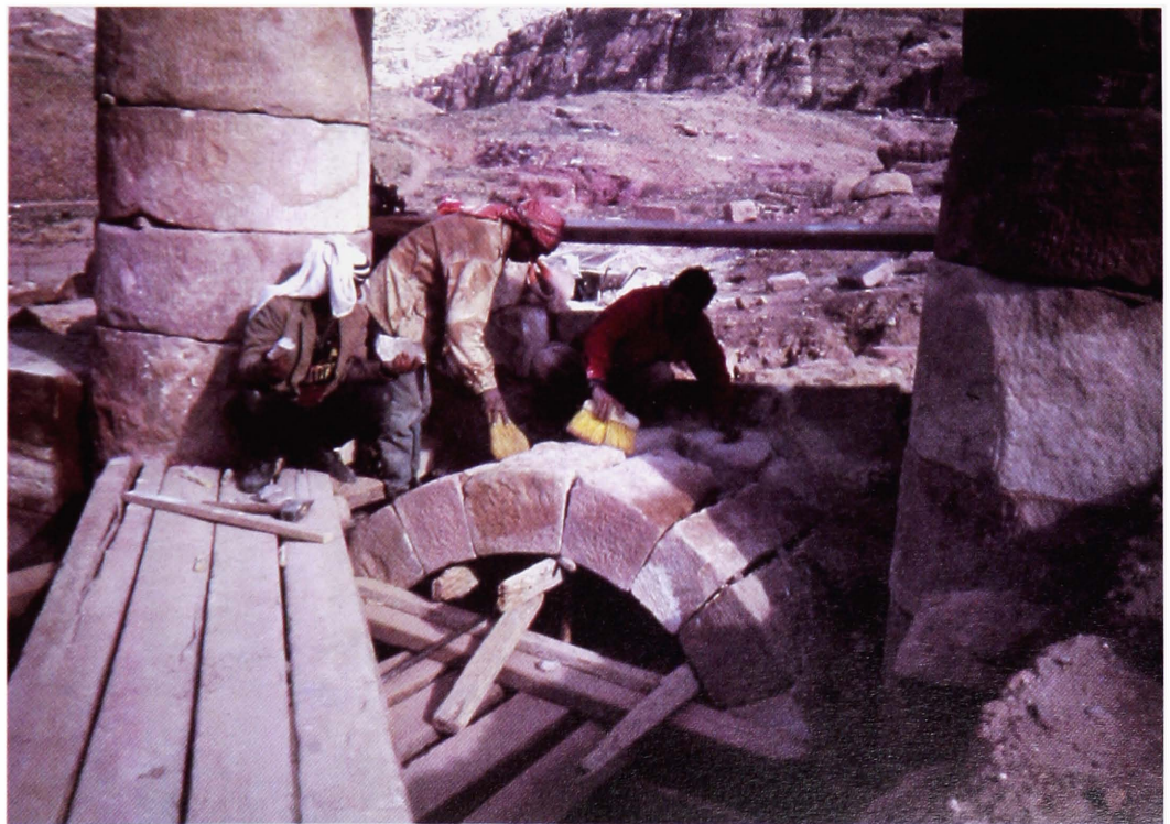
Plates 13, 14 and 15. Anastylis (reconstruction) of the Inter-columnar Wall of the West Corridor, 1997-1998.
