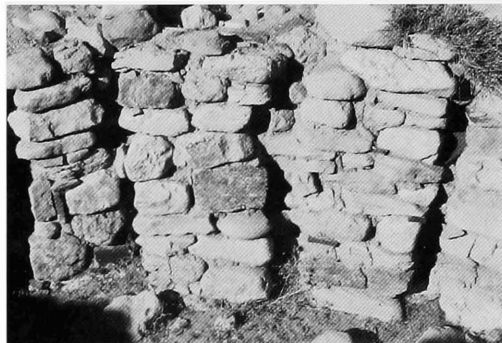
Figure 1.15. Interior wall construction, Al-Bayda'.
