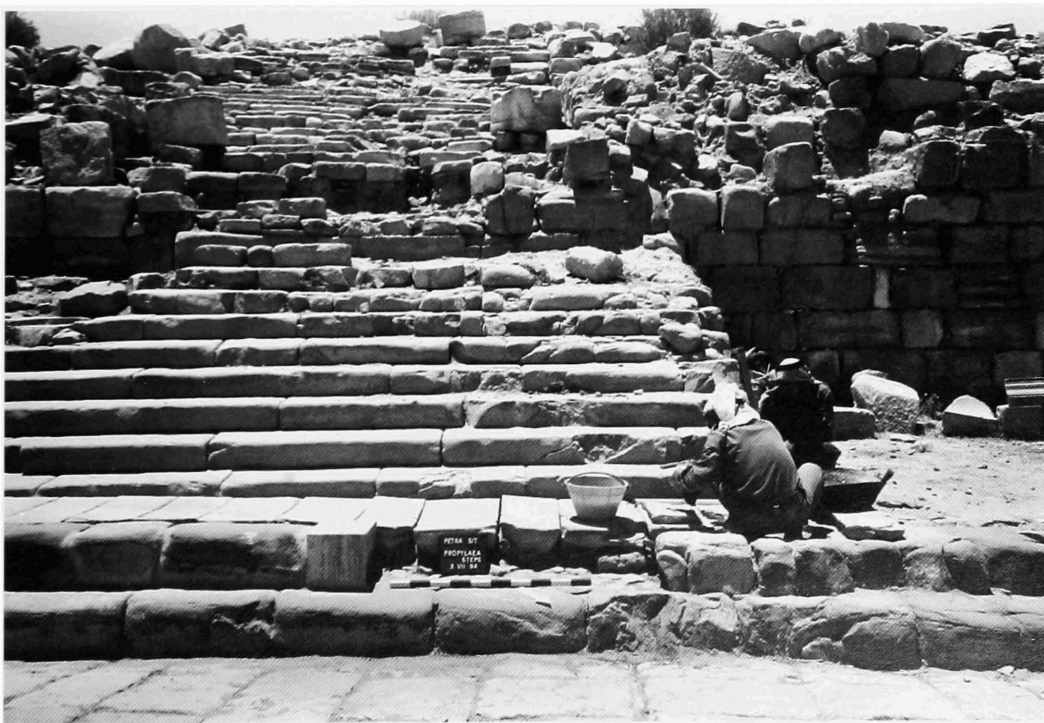
Figure 5.4. Partial consolidation of the Stairs of the Propylaeum.
