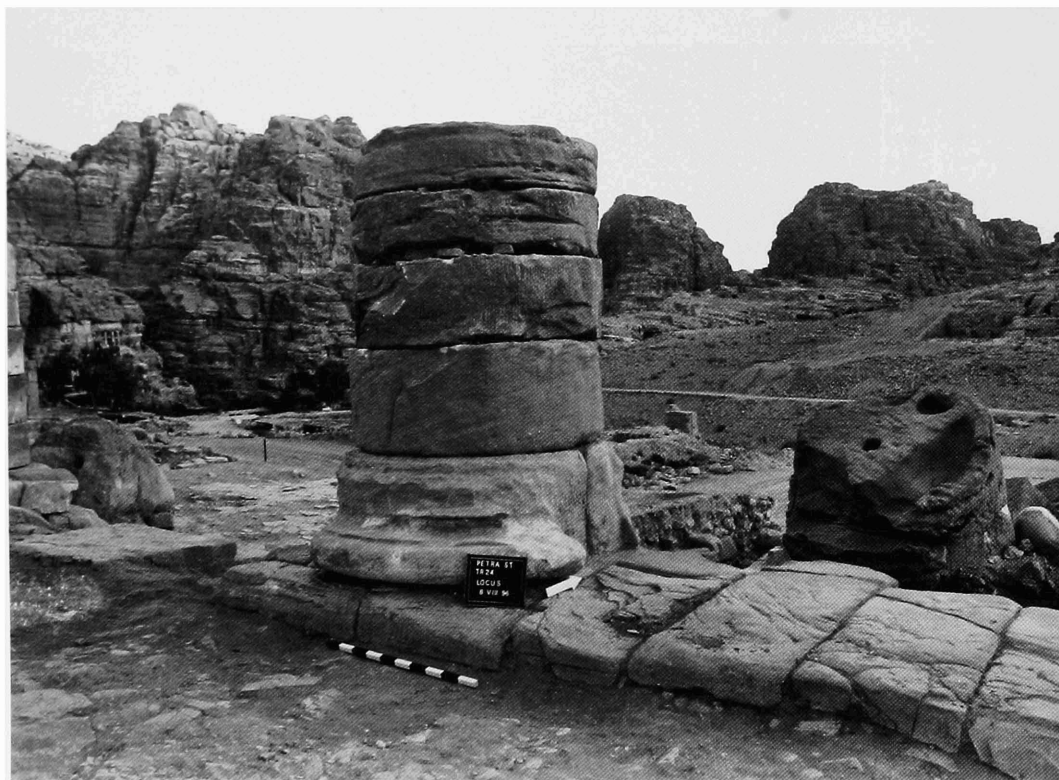
Figure 2.51. Porch column ( Pia Column ), 1996.
