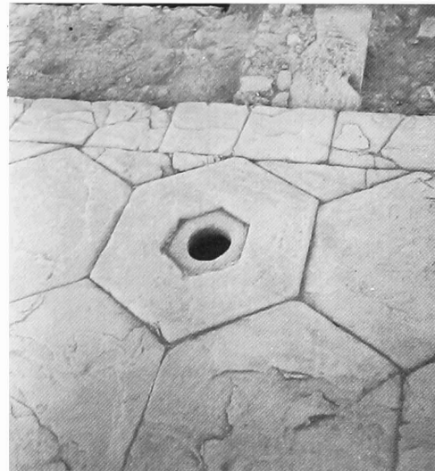
Figure 5.7. Drain, east edge of the Hexagonal Pavement.
