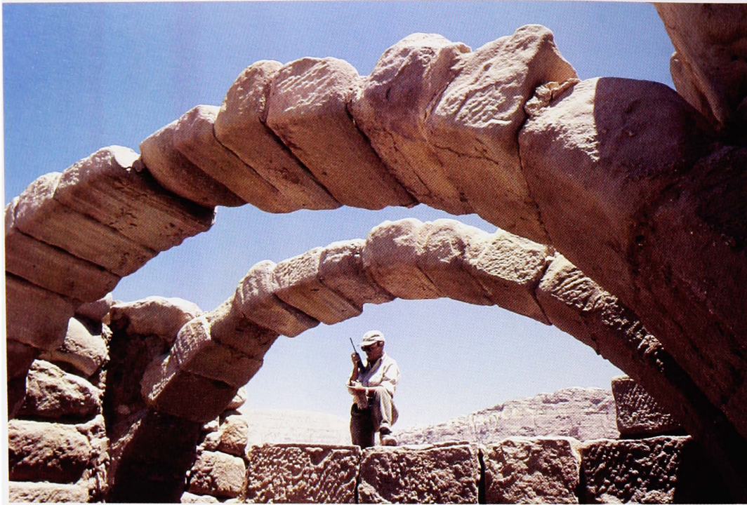
Plate 10. The 'Cistern' arch system. Photograph by John Forasté.
