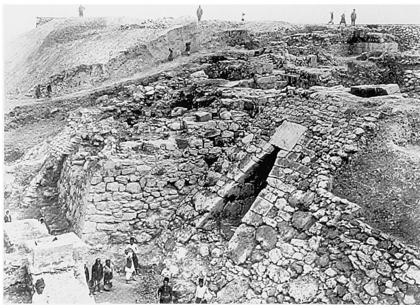
Figure 16. Excavation of the gate and its fortification in 1939, looking north.
