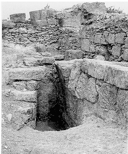
a. The entrance of the sewer, north of the "Royal Plaza," 1984.
