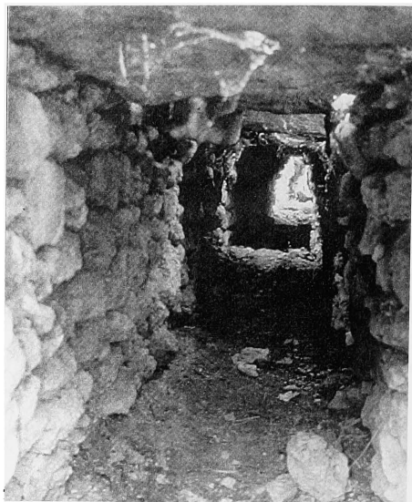
b. The interior of a section of the underground sewer system, in front of the "Queen Mother's Residence," 1986.
