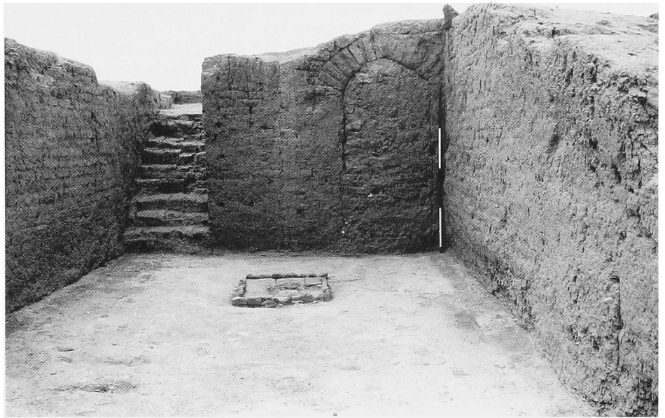
Figure 13. Palace Room 9 from the south, showing the western stair with the vaulted passage beneath, and the brick-built hearth in the centre of the room (see also Fig. 24).
