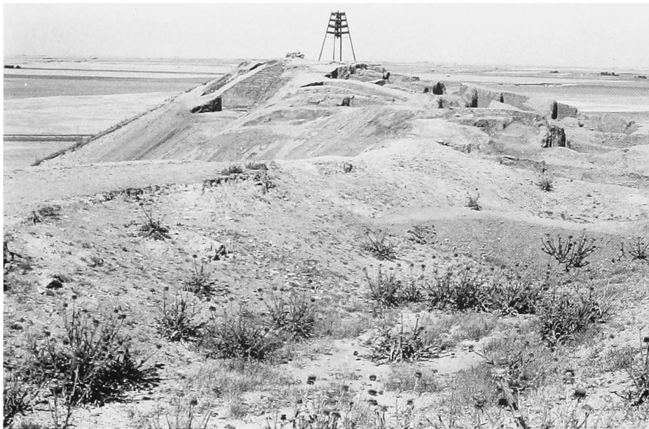
Figure 170. The Mitanni public buildings as revealed at the end of the 1986 excavations, viewed from the west. What survives of the great north reception room (11) can be seen on the left.
