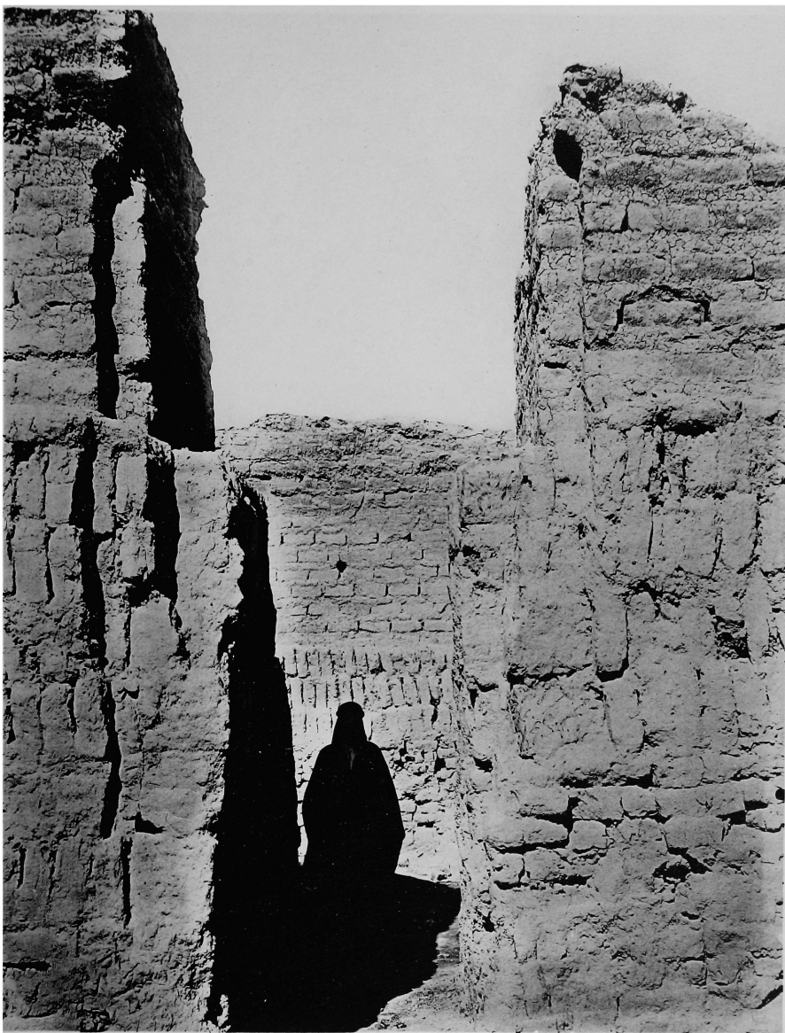
Bricks piled against the walls in the rooms
