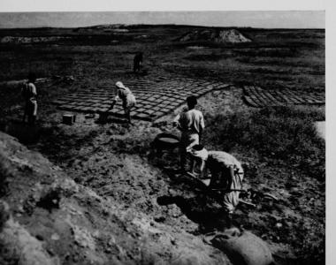
19. Workmen making mud-bricks for an extension to the Expedition house in 1951 (see p. 53). They drew water from a well in the N.W. Palace of Assur-nasir-pal.
