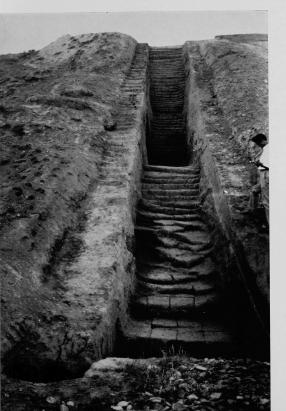
29. Section through east wall of akropolis exposing mud-brick core and footings on external face. Thickness 37 metres. See p. 76.
