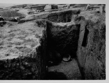
108. Magazine, ZT13 in the north wing of the N.W. Palace. The north wall is built at a slope or batter which helped to support external towers; the recess seen on its inner face served the purpose of a cupboard and its bottom shelf was about 3 ft 6 in above the level of the floor. In the corner a group of pottery as left in about 612 B.C. The whole of this chamber was filled with ash from the destruction. See p. 177.
