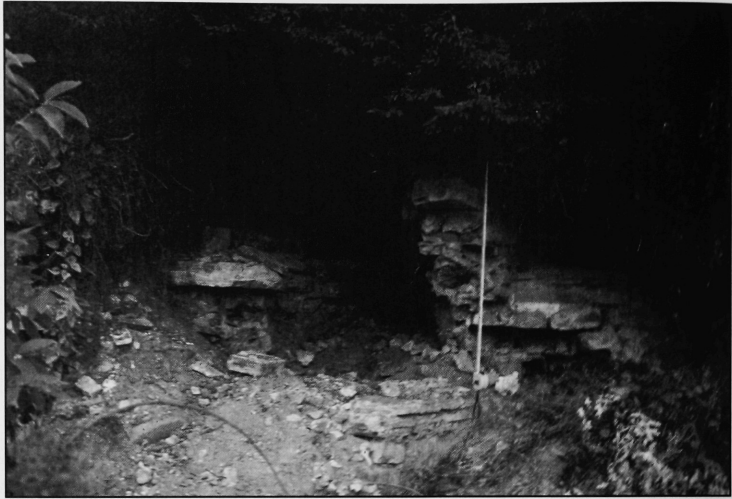
Figure 6-18: Illegal excavations at Kuz mahallesi (Erfelek) have exposed parts of a church structure.
